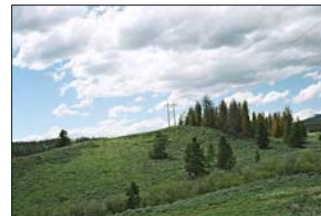
Existing line, southwest of County Road 40
