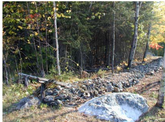
Before repairs—note remnant of fence
