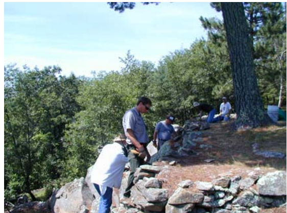
Repairs in progress on same wall
