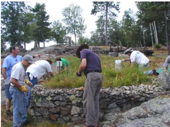
Repairs in progress
