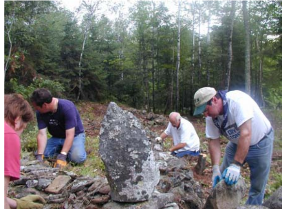
Repairs in progress
