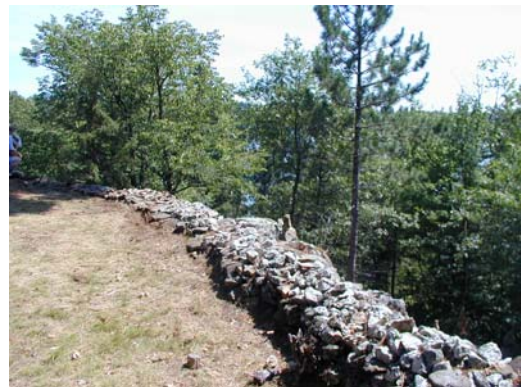
Repaired section of same wall
