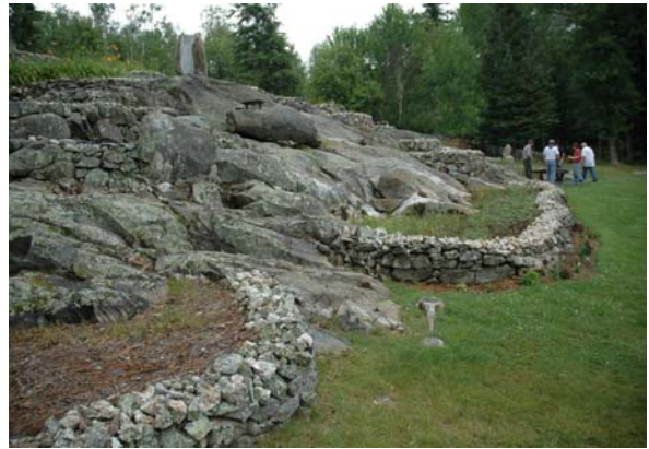
Completed repairs (bed on left)
