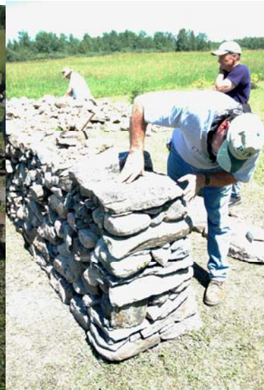
Laying the cover course
