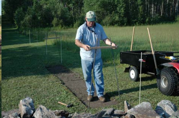
Setting batter frames
