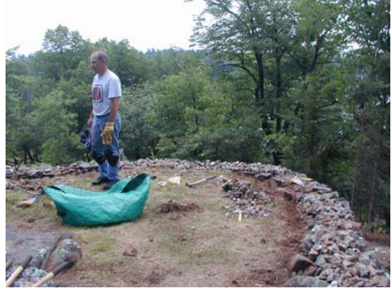
Repaired section of same wall
