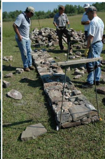
First course completed
