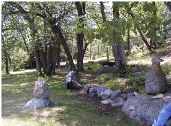
Repairing double boulder wall
