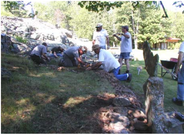
Repairs in progress
