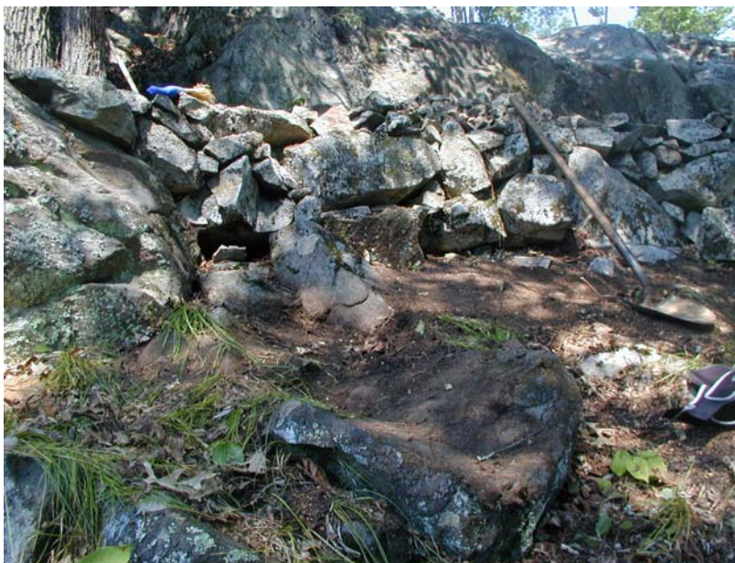
Drainage feature in stone wall
