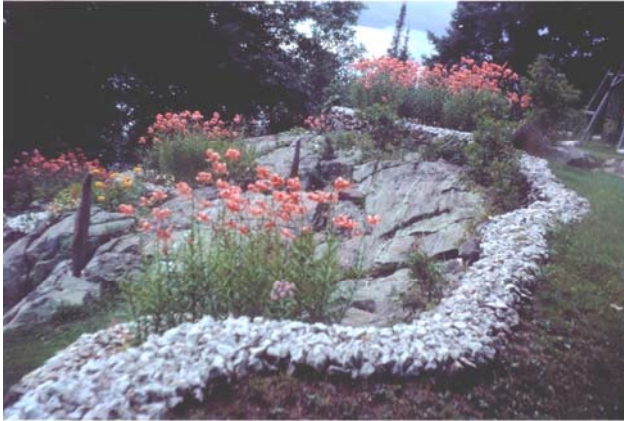
Section of Kabetogama overlook wall ca1963
