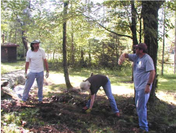
Repairs in progress
