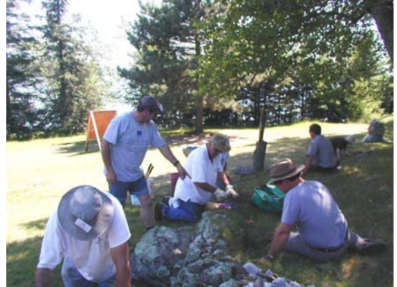
Repairs in progress
