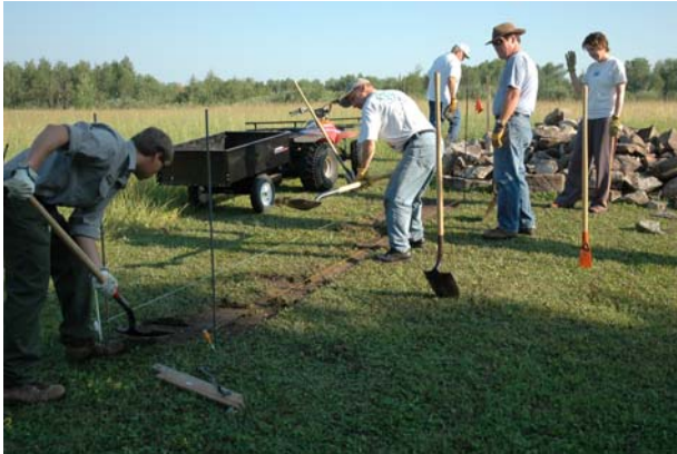
Preparing ground for wall construction
