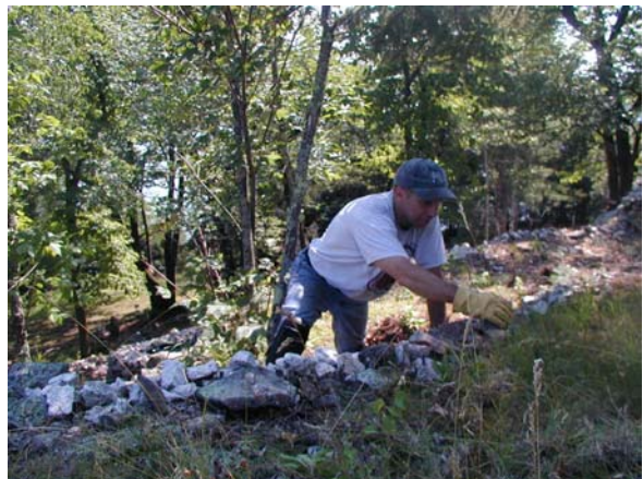
Repairs in progress
