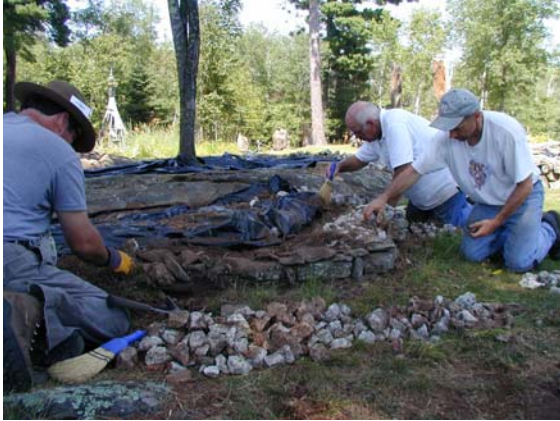
Repairs in progress
