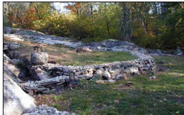
Same wall after repairs in 2006
