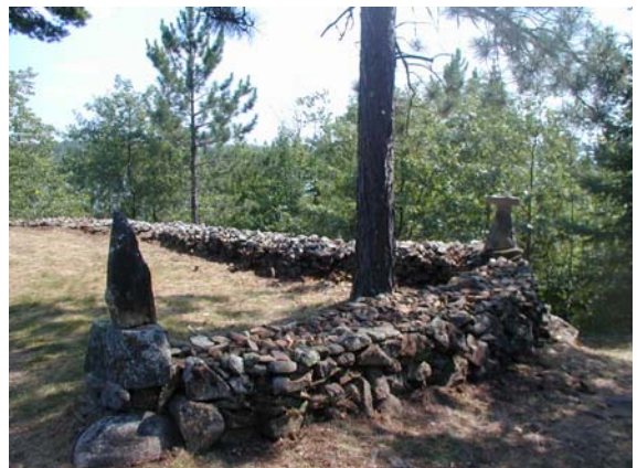
Repaired section of wall
