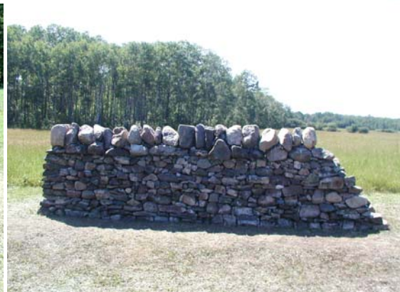
Completed section of wall
