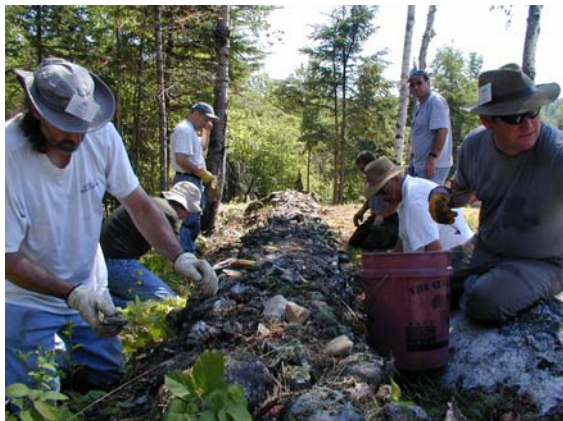
Repairs in progress
