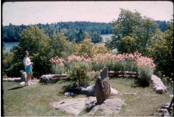
Section of Kabetogama overlook wall ca1961
