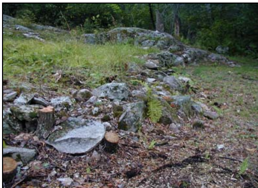
Stone wall before repairs
