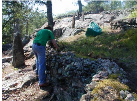
Repairs in progress
