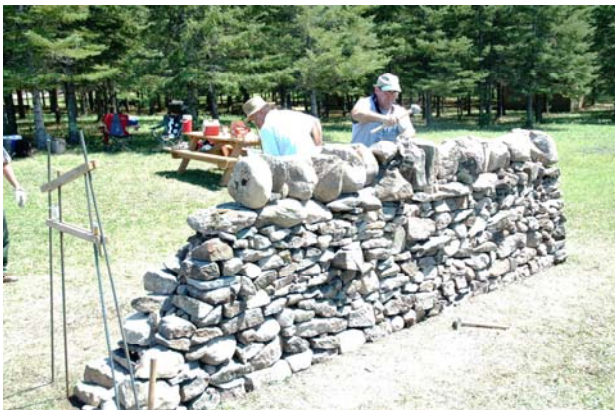
Building the coping layer
