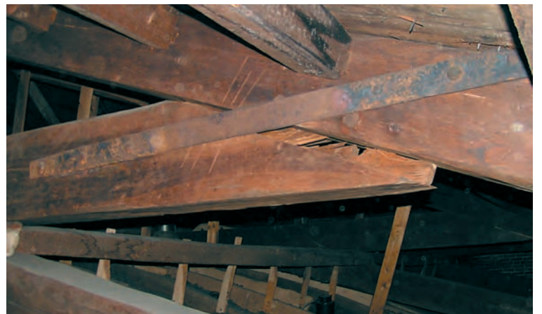
Fig. 29. Tenon destruction in raised chord withdrawn from principal rafter in St. John's truss. Strap may conceal shear failure in chord.
