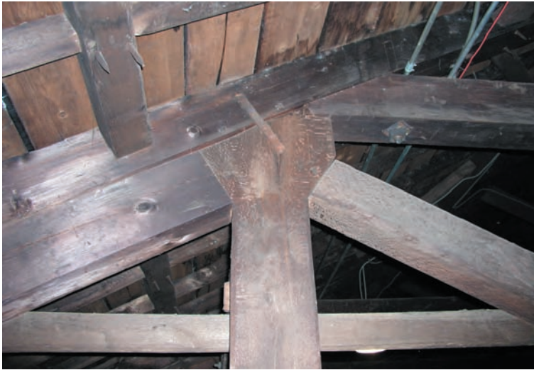
Fig. 8. Some queenpost heads at Central Moravian, obstructed by struts, cannot be bolted to the principal rafters and are stapled instead.
