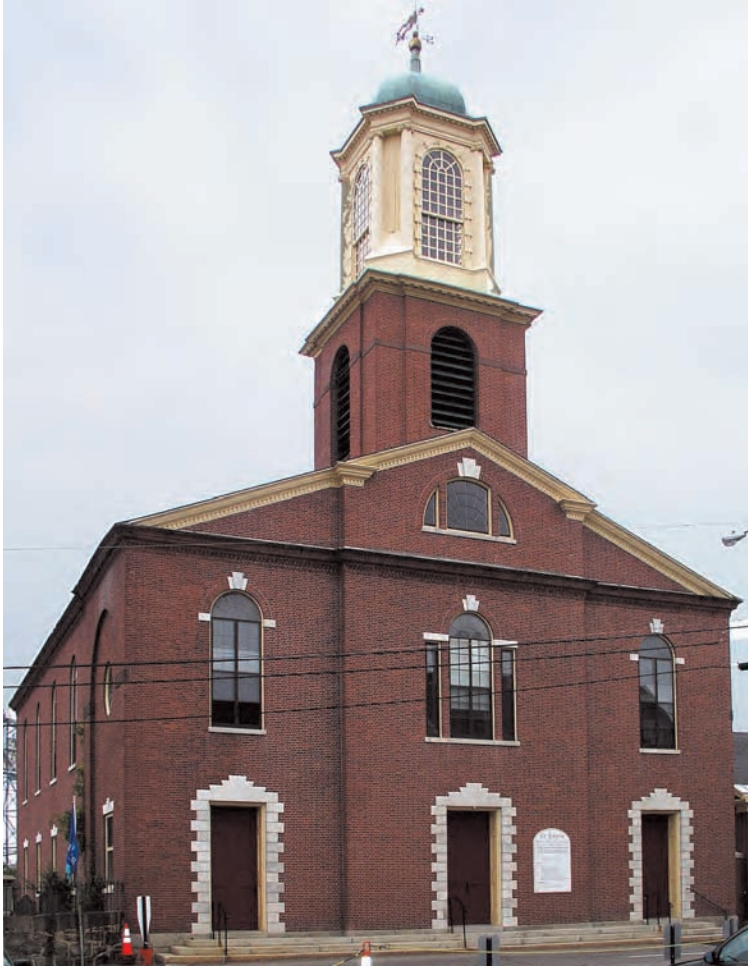
Figs. 26 and 27. St. John's Church, Portsmouth, N.H., 1807, rich in crisp neoclassical detail. The cornice and pediment base are made of molded brick. Below, tapered and carved gallery posts directly support short posts of truss hidden in attic. Researchers in background.
