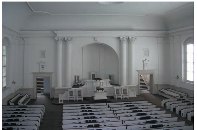
Fig. 11. Coved ceiling is formed entirely below the attic floor. Spacious, classically decorated interior is well maintained.
