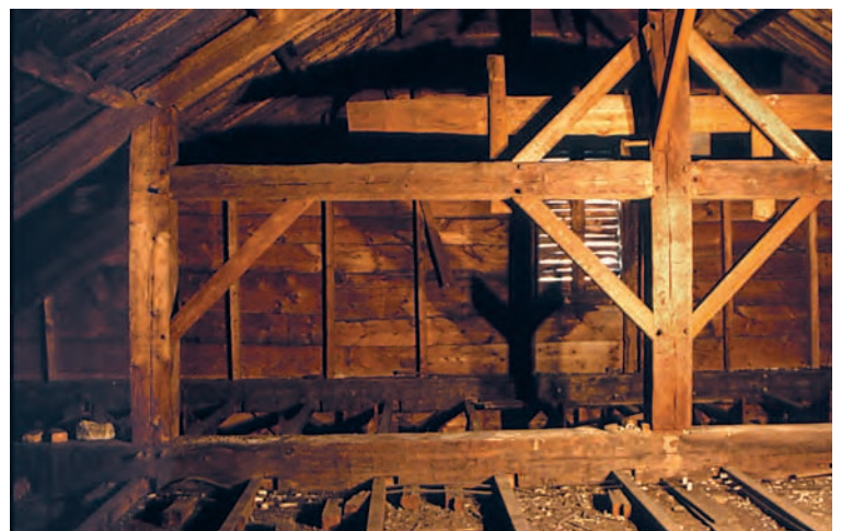
Fig. 3. Naïve truss at Newbury, Vermont, Methodist Church, 1829. Apparent queenpost merely adds unwanted load to truss chord.
