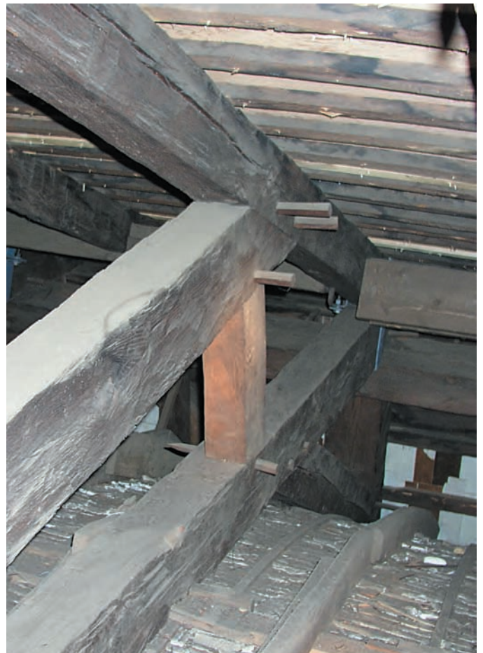
Fig. 22. Principal rafter at Shrewsbury descending past connection with raised chord to meet oblique tie over plate. Brace rises from post to oblique tie, and vertical strut connects latter and raised chord. Some back-primed shingles visible at wall.
