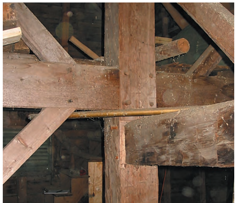
Figs. 33 and 34. Kingpost in tower truss at Sutton Baptist Church is supported by pins at the top and by the tenons of the braced beams seen near bottom of photo and also seen passing from left to right in the photo below. Below, the kingpost is linked and braced back to the bottom of the next kingpost truss via the lowest beam seen on the right.
