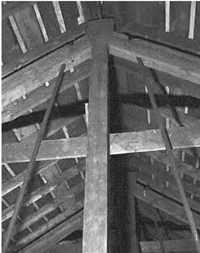
Iron rods support scarfed tie beam. Edge-halved scarf in floor girder. Notch carries joist. Quaker meetinghouse was built for two sexes.
