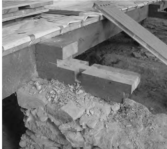
Iron rods support scarfed tie beam. Edge-halved scarf in floor girder. Notch carries joist. Quaker meetinghouse was built for two sexes.
