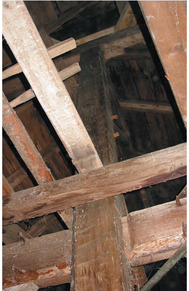
Figs. 33 and 34. Kingpost in tower truss at Sutton Baptist Church is supported by pins at the top and by the tenons of the braced beams seen near bottom of photo and also seen passing from left to right in the photo below. Below, the kingpost is linked and braced back to the bottom of the next kingpost truss via the lowest beam seen on the right.
