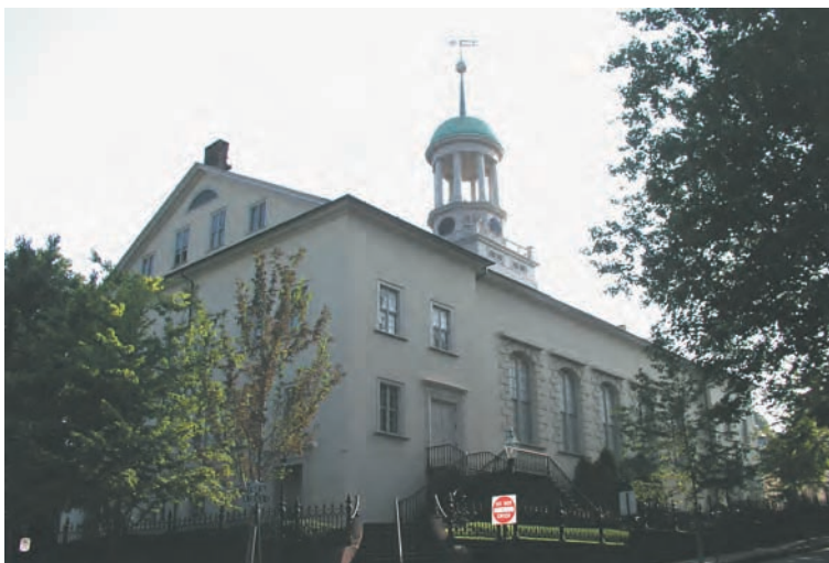
Fig. 9. Rubble stone walls at Central Moravian are parge-d. Substantial cupola is placed centrally, supported ultimately by six trusses.
