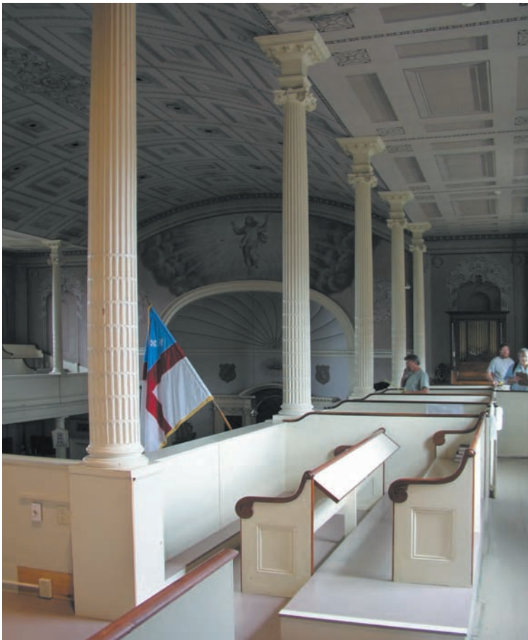
Figs. 26 and 27. St. John's Church, Portsmouth, N.H., 1807, rich in crisp neoclassical detail. The cornice and pediment base are made of molded brick. Below, tapered and carved gallery posts directly support short posts of truss hidden in attic. Researchers in background.
