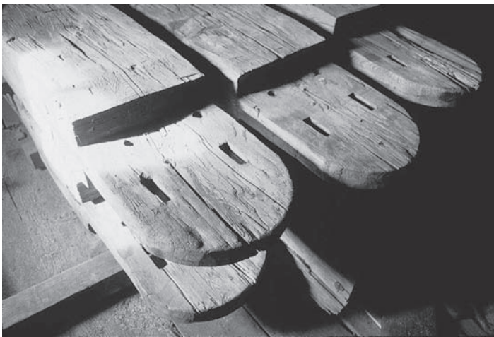
Anchorbeam tenon ends from a pre-1820 Dutch barn taken down in Altamont, New York.
