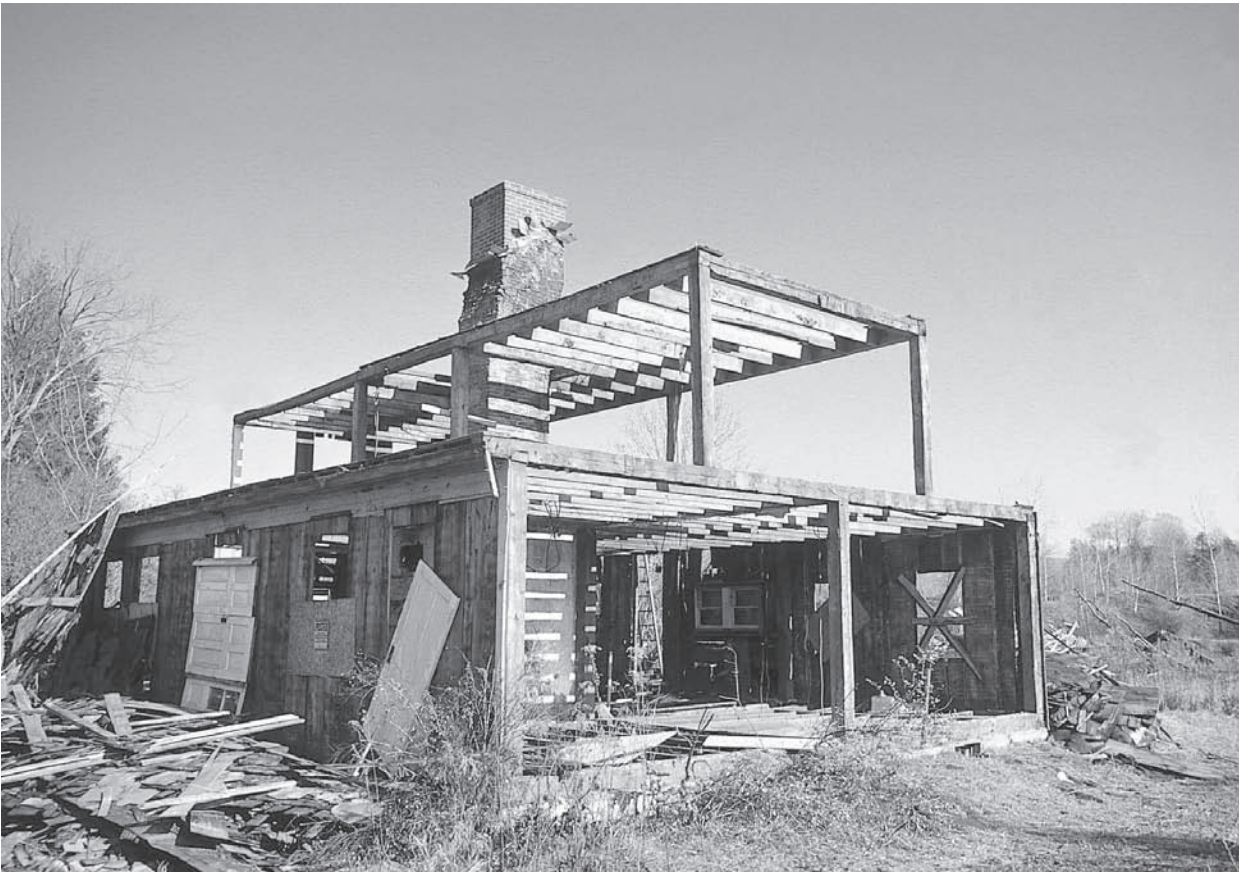
Above, flush tying joints, with top of tie beam and top of plate coplanar, yield neat box frames, as seen in this partly dismantled 1791 house in Cheshire, Massachusetts (see Figs. 11 and 12 of this chapter). Below, mid-18th-century aisled barn in Kensington, New Hampshire, with English tying joint and rare extended tie beams that cross the main, continuous plate and carry the members of an interrupted flying plate tenoned between them. The flying plate, seen to the right of the peg, supports a Greek Revival cornice.
