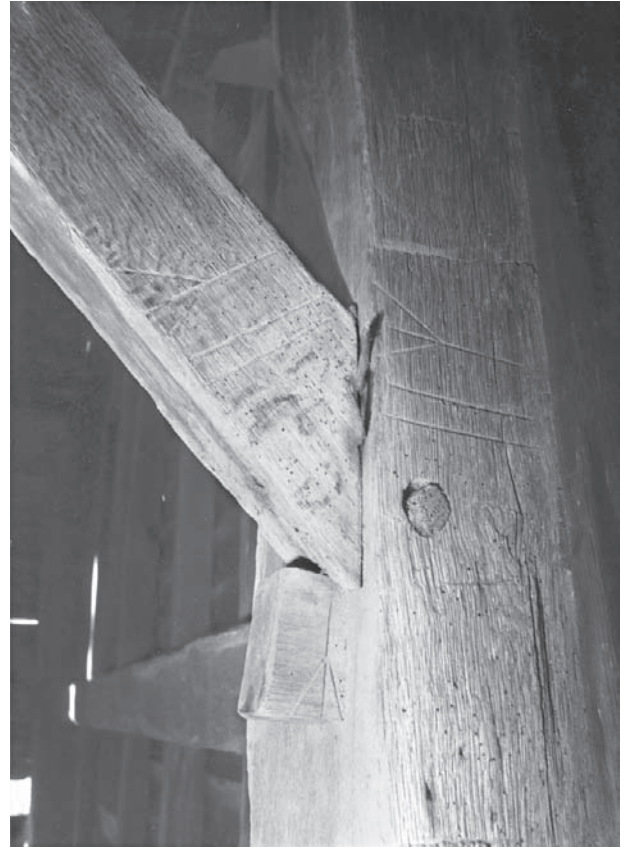
Scribe rule barn in Chatham, N.Y., with packing or distance piece driven to take up space needed to fit brace into made-up assembly of post and beam. Brace, post and packing piece are all marked for reassembly after scribing.
