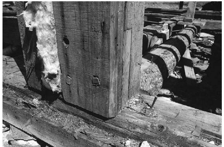
A free tenon in the bottom of a post in this house in Windsor, Mass., may be a repair or a fix for a mistake. Shadows are cast by joists above.
