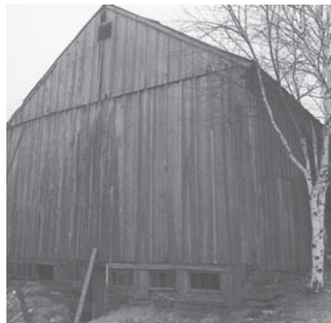
Boarding lapped at tie beam.
