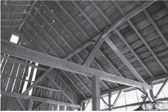
Mid-19th-century Hinsdale, Massachusetts, barn before dismantling. The continuous purlin plate assembly is canted perpendicular to the roof, and the purlin plate is flush with the roof. The rafters tenon into both upper and lower faces of the purlin plate.
