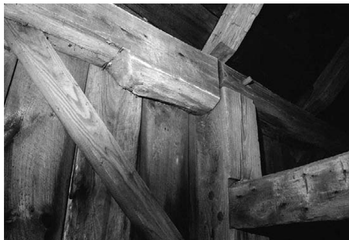
Jowled plate (one of six!) in a much-expanded 18th-century English-style barn, Huntington, Massachusetts.
