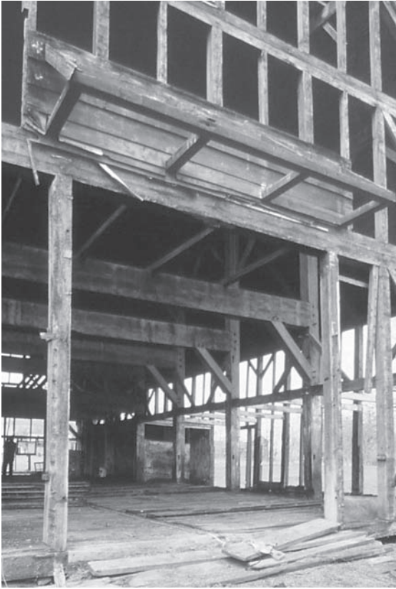
Cantilevered pentice arms run over the end anchorbeam of this Dutch barn formerly in Middleburgh, New York, and support the pentice plate with blind tenons. Rafters are butted and nailed as in Fig. 40.
