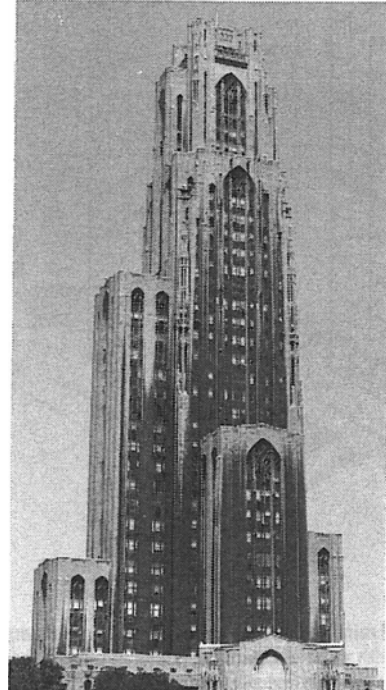
Forbes Avenue Side (facing SE)
