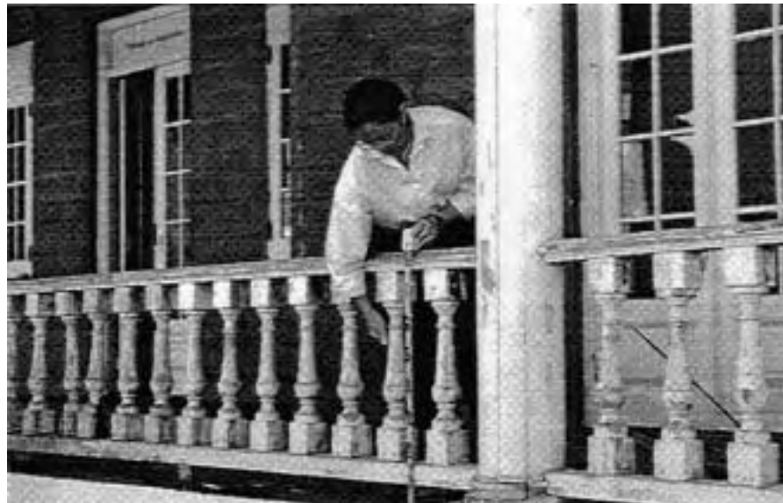
Colegio de Arquitectos Headquarters Inspection work (1993)
