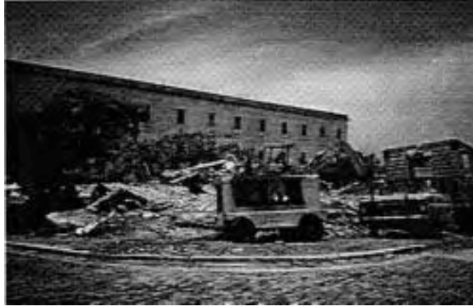
Demolition of existing structures for Plaza Quinto Centenario in Ballajá District of Old San Juan, PR (1986).
