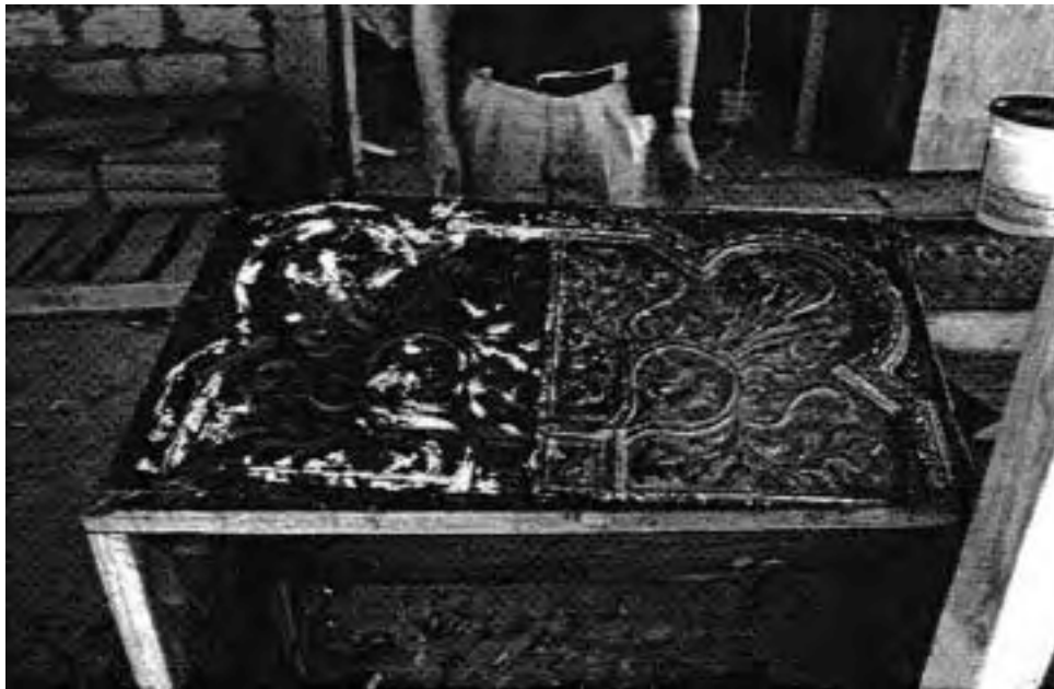
Original (left) and fiberglass reproduction (right) of tin ceiling panels. The original historic examples in good condition were used as molds where replacement panels were needed. Colegio de Arquitectos de Rico Rehabilitation Project (1992).
