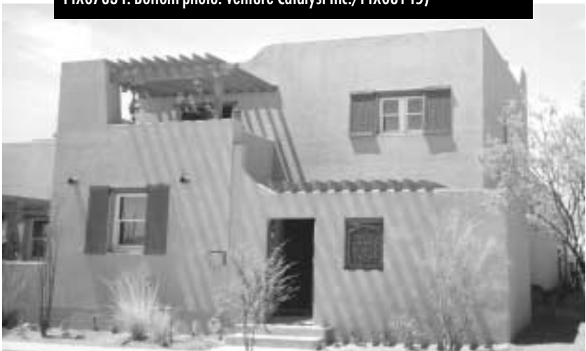
Civano, an energy-efficient community in Tucson, includes a neighborhood center equipped with a 6-kW photovoltaic installation. Each home at the Civano Development in Tucson, Arizona, is 30–60% more energy efficient than the typical, standard construction. (Top photo: George James/PIX07634. Bottom photo: Venture Catalyst Inc./PIX08145)
