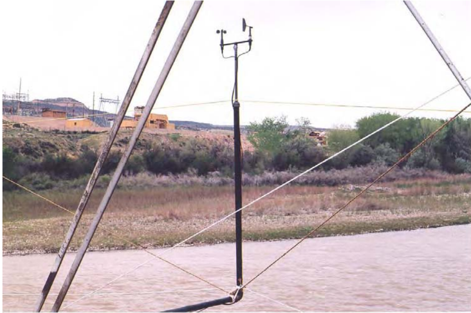
Figure A.7. Anemometer (WS1) and Wind Direction sensor (WD) installed at Fruita Bridge. They are located directly upwind of the centroid of the wind intercept area of the bridge.
