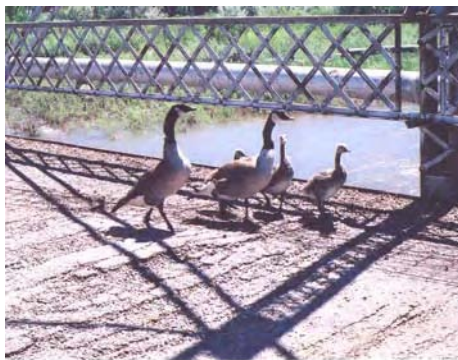
Figure 1.13. Rifle Bridge deck. The deck of (weathered) asphalt pavement on corrugated bridge deck on a combination of steel and timber stringers is similar to that of the Prowers Bridge.
