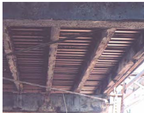
Figure 1.13. Rifle Bridge deck. The deck of (weathered) asphalt pavement on corrugated bridge deck on a combination of steel and timber stringers is similar to that of the Prowers Bridge.
