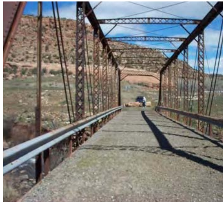
Figure 1.10. San Miguel Bridge Deck. The deck, believed to have been installed in 1964, consists of gravel roadbase on semi-circular corrugated metal pipe segments which bear on the bottom flanges of steel stringers. The metal pipe has been replaced with timber blocks in a few places where the corrugated metal pipe has rusted away.
