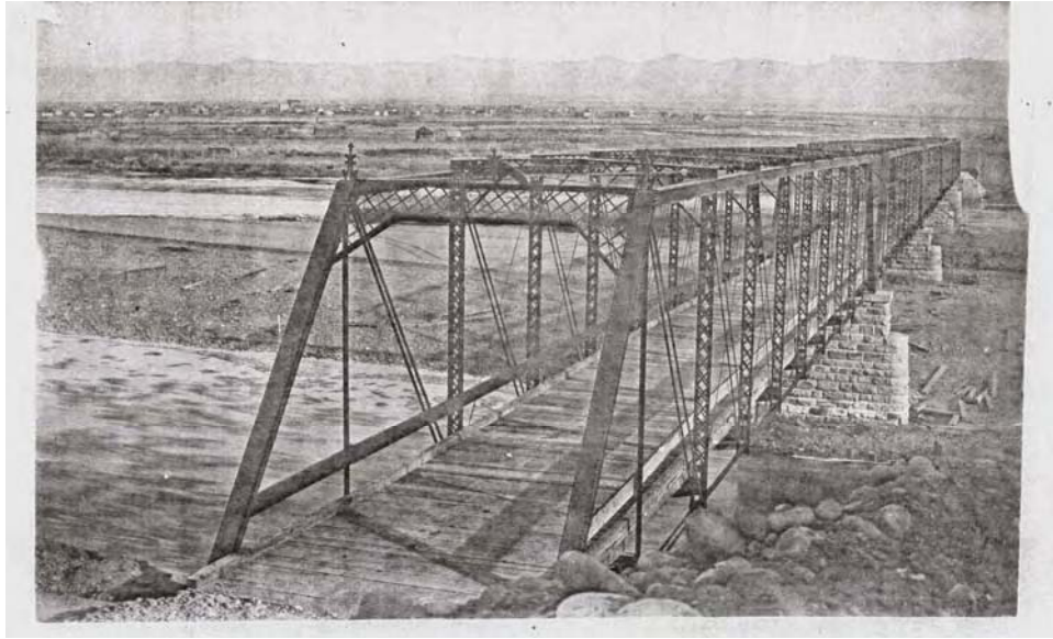
Figure 1.11. Fifth Street Bridge over Grand River, Grand Junction, CO. Built in 1886, this Pratt truss was of wrought iron construction. One span of this bridge was relocated to the San Miguel location in the 1930's. Note the timber deck and very simple, single board railing. (Photo courtesy of Museum of Western Colorado).
