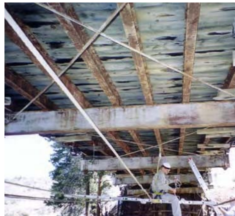
Figure 1.8. Blue River Bridge Deck. The deck consists of longitudinal “running boards” on transverse timbers on steel stringers. The orthogonal criss-crossing of running boards and deck timbers creates a much more continuous deck than that at Fruita Bridge. The steel stringers bear on and are mechanically attached to the steel floor beams.
