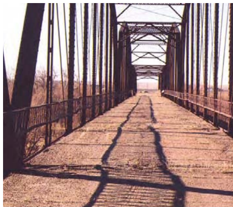
Figure 1.6. Prowers Bridge Deck. The steel stringers are riveted to the floor beams, suggesting that the stringers are original. However, the corrugated bridge deck is clearly a replacement. Asphalt pavement, now significantly weathered, was installed over the corrugated deck.
