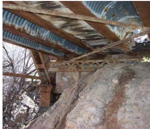
Figure 1.10. San Miguel Bridge Deck. The deck, believed to have been installed in 1964, consists of gravel roadbase on semi-circular corrugated metal pipe segments which bear on the bottom flanges of steel stringers. The metal pipe has been replaced with timber blocks in a few places where the corrugated metal pipe has rusted away.
