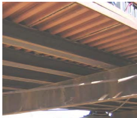
Figure 1.6. Prowers Bridge Deck. The steel stringers are riveted to the floor beams, suggesting that the stringers are original. However, the corrugated bridge deck is clearly a replacement. Asphalt pavement, now significantly weathered, was installed over the corrugated deck.
