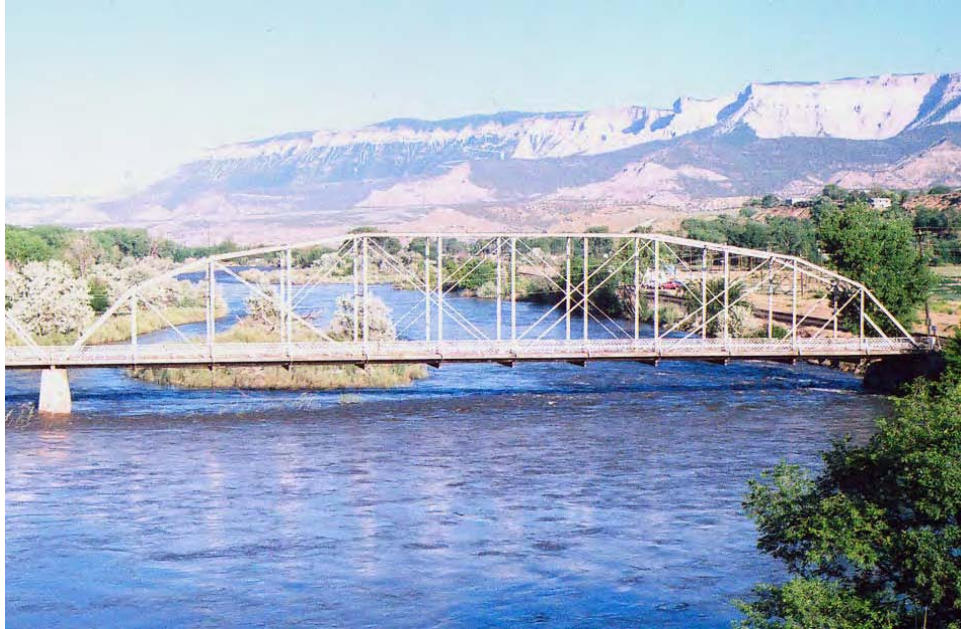
Figure 1.12. Rifle Bridge over the Colorado River at Rifle, Colorado. This 73 meter (240-foot) span Pennsylvania truss comprises the longer of two different spans at that location. It has steel floor beams with steel stringers, covered by a corrugated metal deck with asphalt pavement. It has steel eyebar bottom chords and diagonals and steel rod counterbracing. The railing is a steel lattice with double angle top and bottom rails. It has been abandoned since the late 1960's, when a replacement bridge was constructed.
