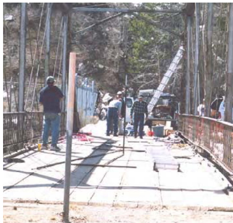
Figure 1.8. Blue River Bridge Deck. The deck consists of longitudinal “running boards” on transverse timbers on steel stringers. The orthogonal criss-crossing of running boards and deck timbers creates a much more continuous deck than that at Fruita Bridge. The steel stringers bear on and are mechanically attached to the steel floor beams.
