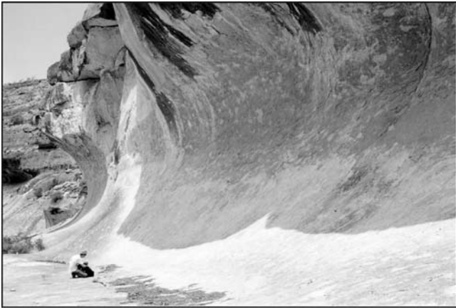
Fig. 2. Photograph showing a typical rock overhang. The rock surface protected from rain and runoff under the overhang is completely covered by the yellowish-brown calcium oxalate coating, while a dark stain (black) occurs on surfaces exposed to rain and runoff.
