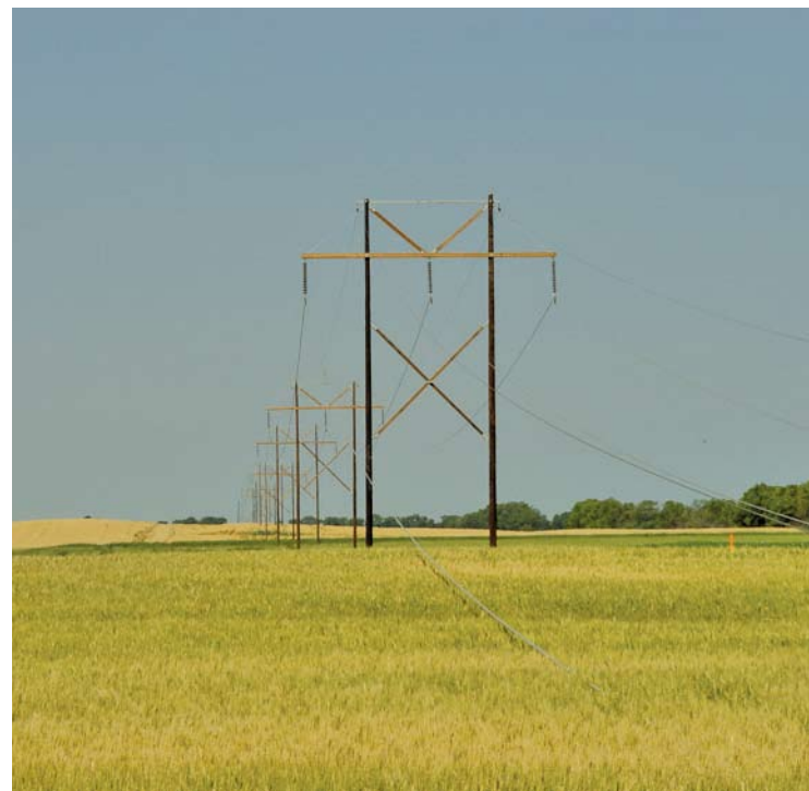
Below: After the July 15 storm mangled 28 steel structures on the Jamestown-to-Fargo, No. 1 230-kV transmission line, Western line crews installed 47 temporary wooden structures to get the line back in service.
