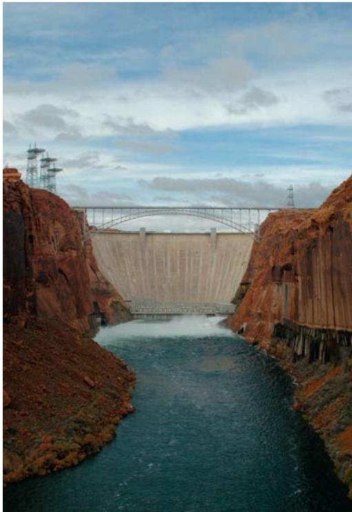
Glen Canyon Dam
