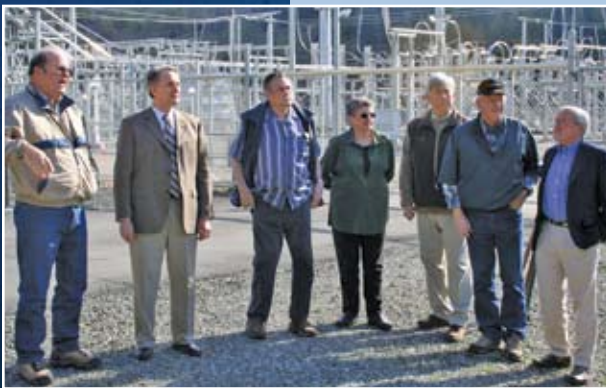
The Trinity Public Utilities Board stands in the Trinity Substation yard. Board member Rick Morris, far right, who has served on the board since the utility's inception, has waited to see the substation built since 1955.
