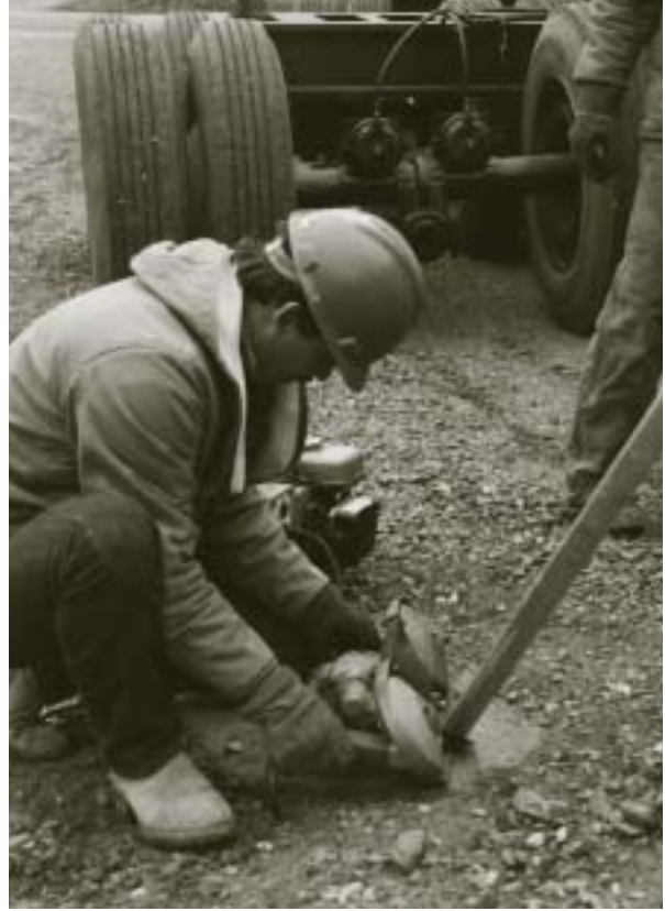
Crews prepare the Olinda Substation (later renamed for Congressman Vic Fazio) for the arrival of the first transformer.
