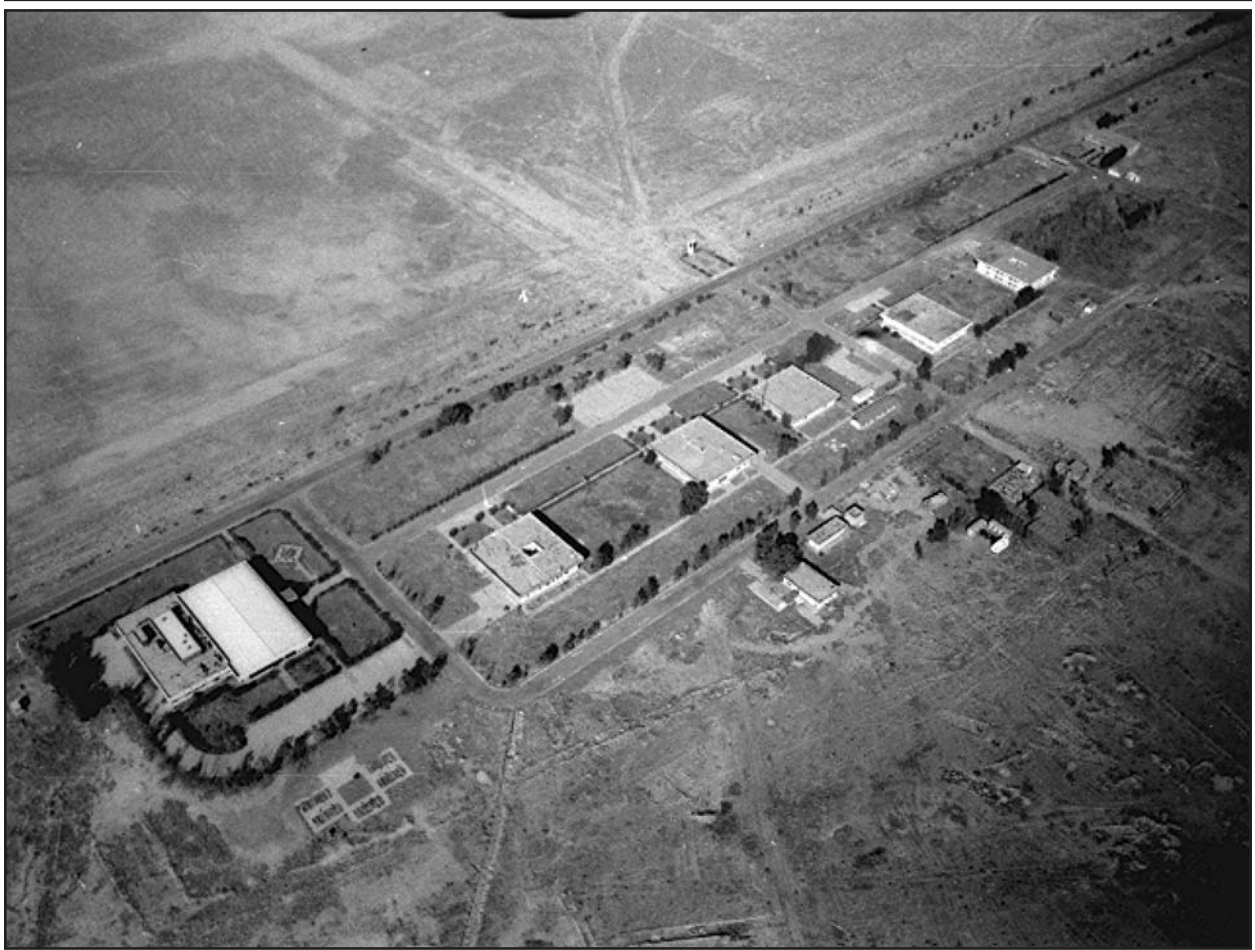
Figure 8. Al Muthanna administration support area razed after 1994.
