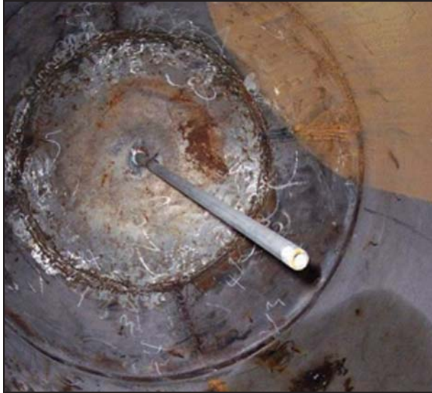
Figure 6. The inside of the reactor vessel on trailer 2.
