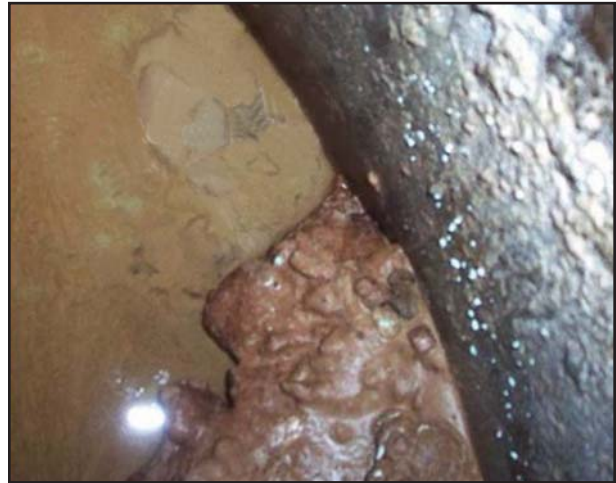
Figure 8. Solids in the bottom of the reactor vessel on trailer 1.
