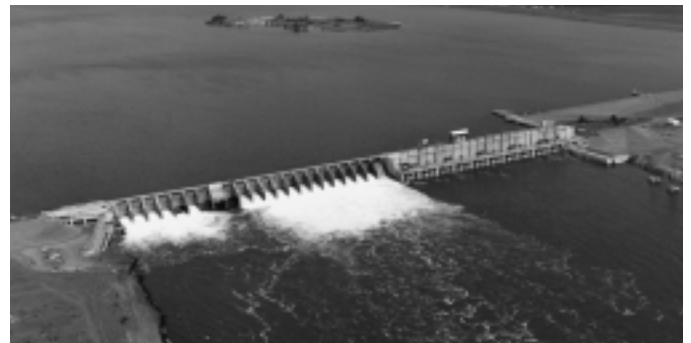
The Council has worked to improve consideration of historic properties for hydropower relicensing projects and Historic Resources Management Plans at hydroelectric facilities. Priest Rapids Dam in Washington State is one such example. (Photo courtesy of Grant County Public Utility District)
