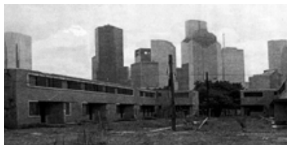
Allen Parkway Village, a circa 1941 public housing complex in Houston, before it was revitalized using HUD monies.
