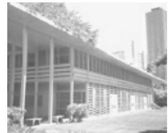
Maluhia Hall, or "haven of rest," at Fort DeRussy in Honolulu, Hawaii, featured wood-louvered doors and decorative cut-out panels depicting island motifs.
