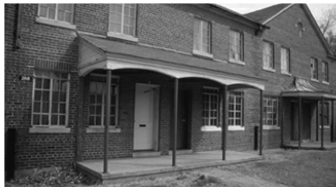
Built in 1938, Lauderdale Courts, a public housing complex in Memphis, Tennessee, is in poor condition, but the overall site plan retains its historic features. (Photo courtesy of Memphis Explorations, Tennessee)
