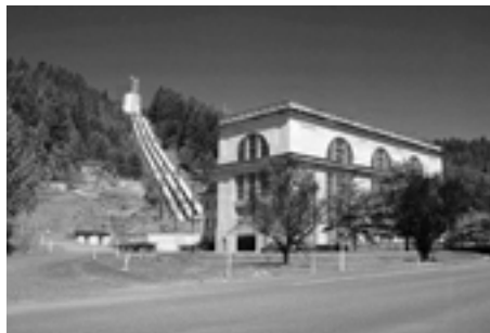
Penstocks are diverting water from the North Fork Skokomish River to Cushman Powerhouse No. 2. (Photo courtesy of Tacoma Public Utilities)
