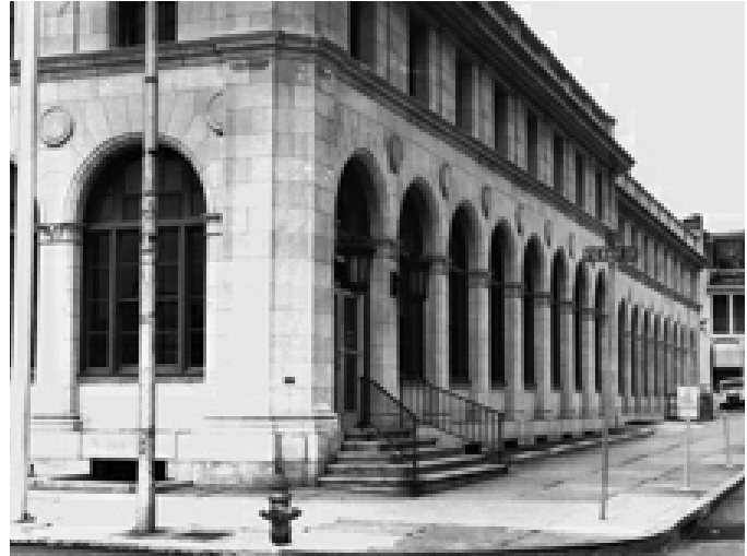
Representative of small-town Federal Government architecture at its best, Easton, Pennsylvania's, Main Post Office was slated for demolition. Citizens used the Section 106 review process to persuade the Postal Service to opt for rehabilitation.
