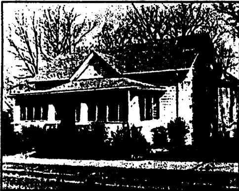
An enclosed front porch, compromises the historic character of the house and streetscape.
