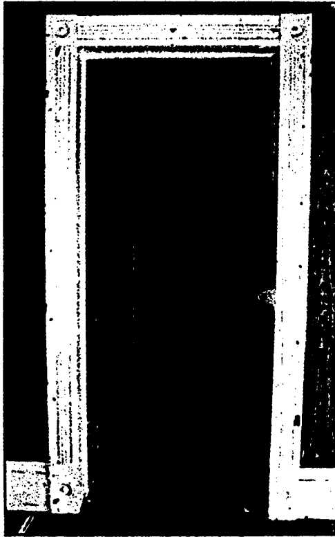
Distinctive moldings and corner blocks like these should be preserved when possible.
