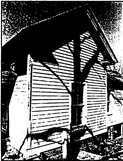
Here, deteriorated wood clapboards were replaced with fiber-reinforced cement siding to match their size and spacing. The wood trim was retained.
