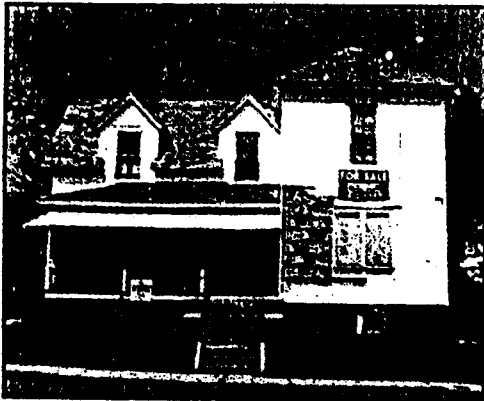
The wood clapboards on this house had been covered first in asphalt shingles and then vinyl siding. Since the vinyl siding was intact except for the small area seen on the front wall, the vinyl was repaired and retained.
