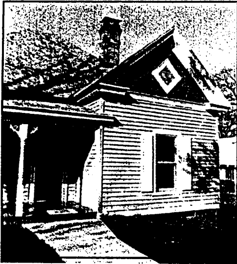
The wood clapboards on this house had been covered by asphalt shingles earlier. Vinyl siding was installed over the asphalt shingles, but the wood shingles in the front gable and the original trimwork were retained and repaired.
