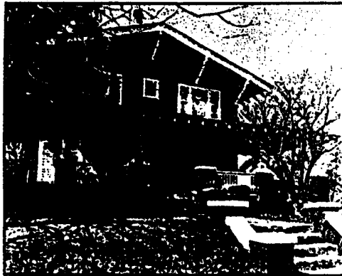
Projecting brackets and exposed rafters like those found on this bungalow are distinctive exterior trimwork features that should be retained.
