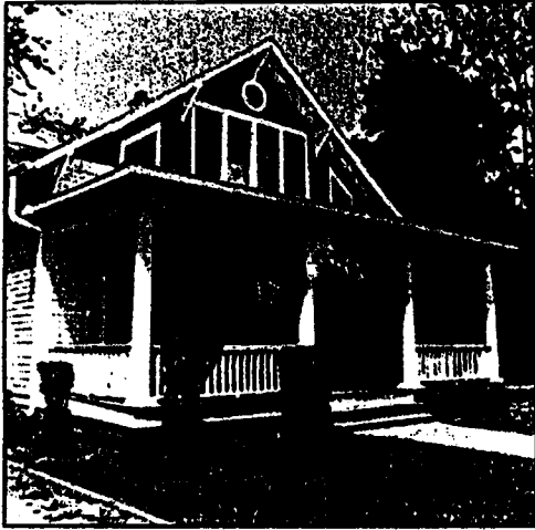
Craftsman style elements such as the exposed gable brackets and the wood shingles in the front gable embellish many of the early twentieth century bungalows, like this one, in the historic district.
