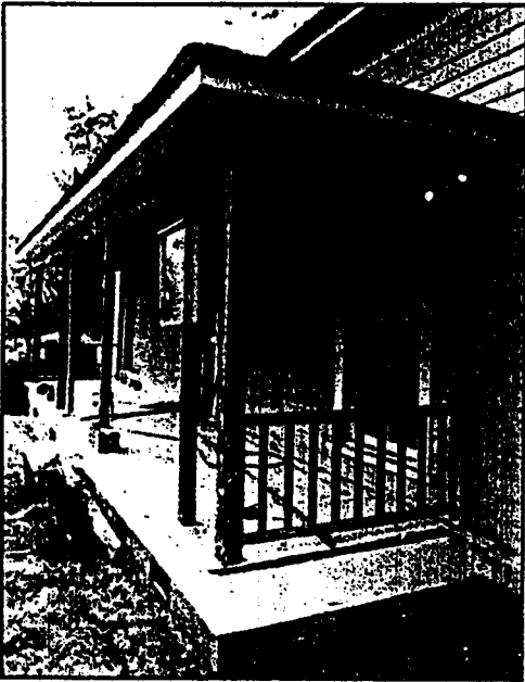
To save costs, compatible replacement railings will be used between the original porch columns which were repaired and stripped of lead paint.
