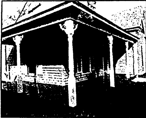
This porch rehabilitation involved various options: the turned columns, cornice, and beaded board ceiling were repaired, the floor was replaced, and only a single missing bracket was special ordered.
