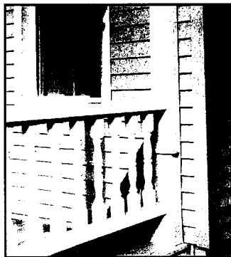
A fairly careful use of vinyl siding is evidenced on this Beers Street house. Careful attention was paid to corner boards and window casings.
