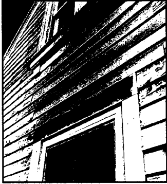
Often original siding is in surprisingly good condition. Over a century of service is a tribute to the durability of the material. Repairs frequently consist of the replacement of a few individual clapboards (seen here as the smooth boards above the window).
