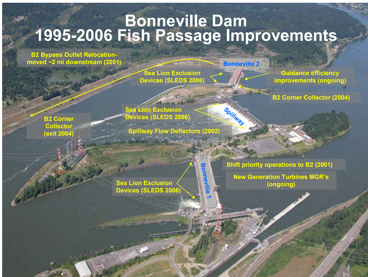
Figure A-4. Improvements at Bonneville Dam from 1995 to 2006
