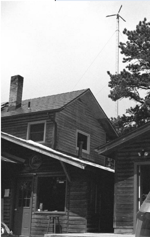
Jim Green, NREL / FTX02796
