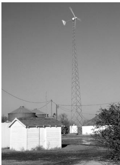
Warren Gretz, NREL/PT09634
