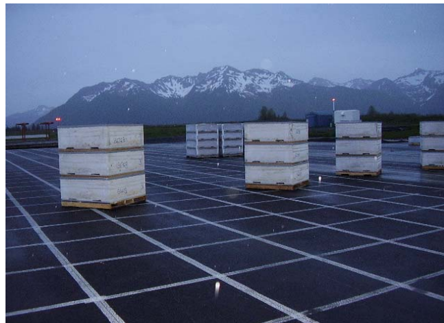
Cordova, AK EMAS (Engineered Material Arresting System) block laying in progress-June 2007
