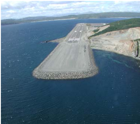
Sand Point, AK RSA under construction 05
