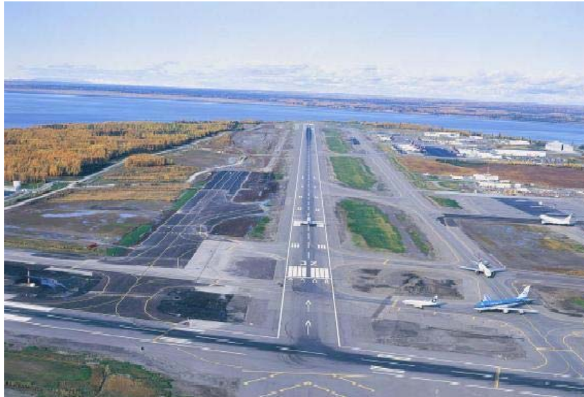
Ted Stevens Anchorage International Airport, N/S taxiway construction, 2004
