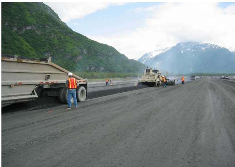
Valdez Airport Runway Reconstruction, 2006
