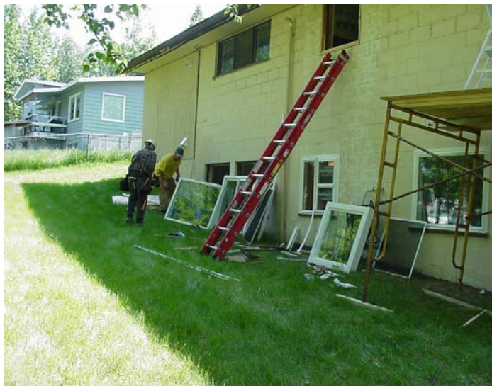
Ted Stevens Anchorage International Airport, Residential Sound Insulation Program
