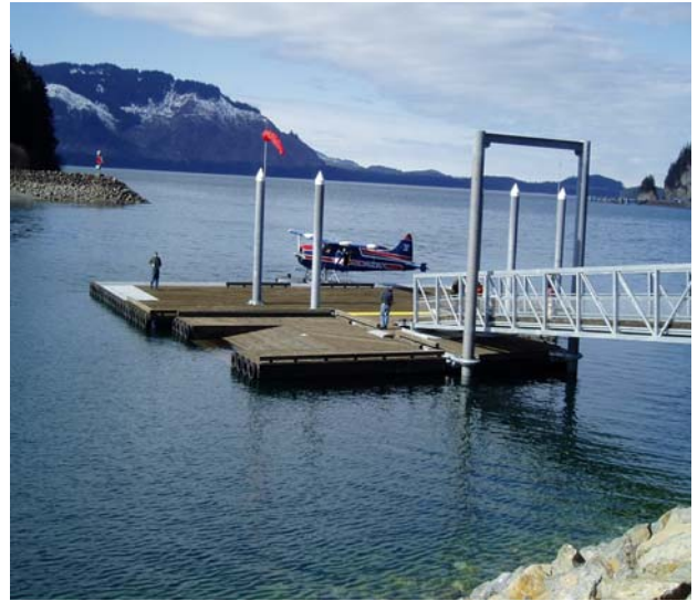
Hoonah –New SPB completed
