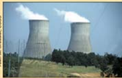
Cooling towers, Burke County, Georgia
