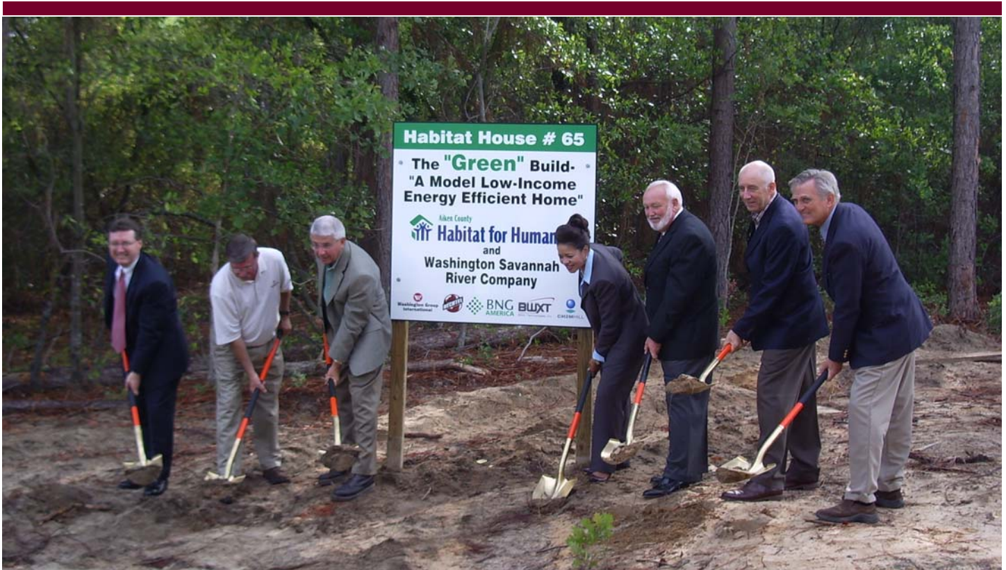
Breaking ground are from left, Keith Wood (WSRC Director of Public Affairs); Chuck Campbell (WSRC Habitat Green Build Project Lead); Bill Poulson (WSRC Executive Vice President for M&O); Lessie Price (WSRC Manager, Community Assistance); Ronnie Young (Chairman, Aiken County Council); Jack DeVine (WSRC Senior Advisor and Aiken County Habitat for Humanity Board Member); and Richard Church (Executive Director, Aiken County Habitat for Humanity)
