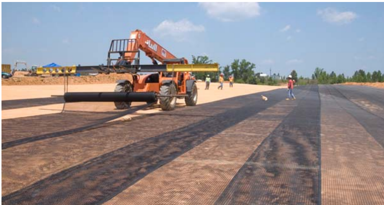
Installation of the geosynthetic cover
