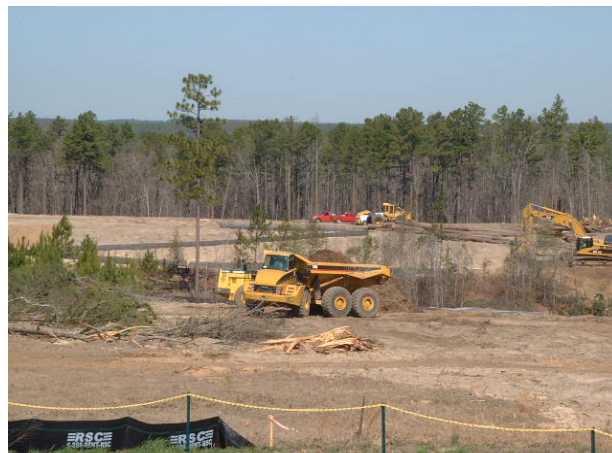
Preparing the site
