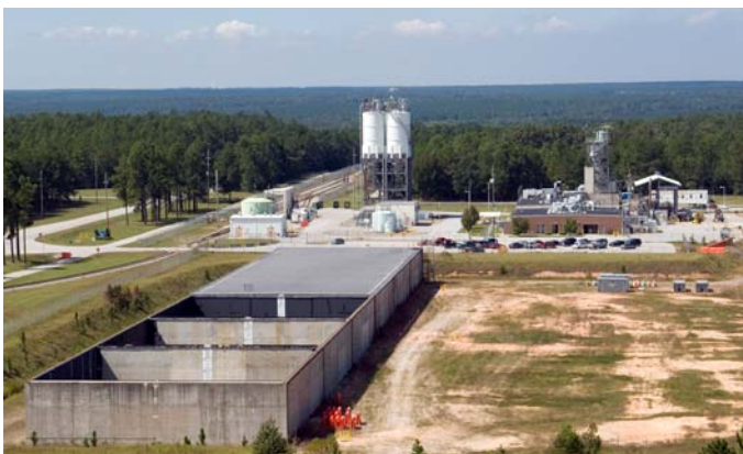
Saltstone Facility in Z Area
