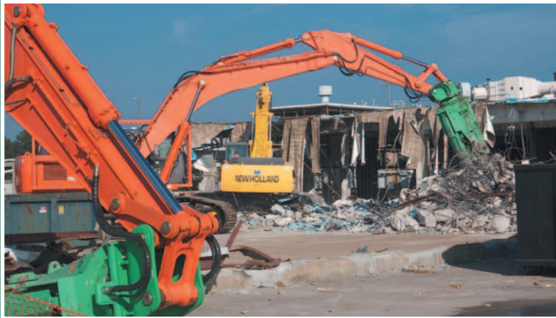
▲ One of the more than 160 buildings being demolished on site.
