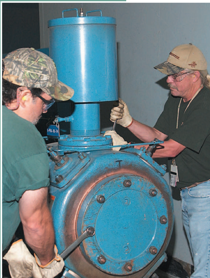
▲ F Canyon employees perform deactivation work on equipment inside the canyon.
