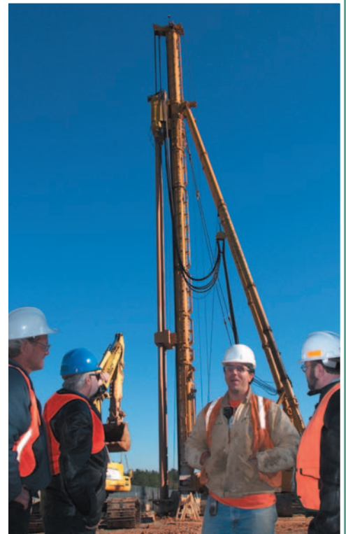
▲ Barrier walls have been installed in F and H areas to slow the migration of contaminants.
