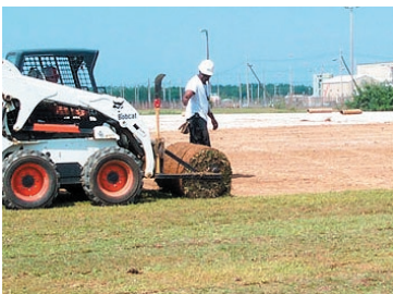
▲ Sodding work is conducted at a remediation site.
