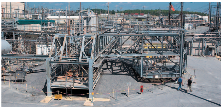
▲ A view of the F Area Tank Farm.
