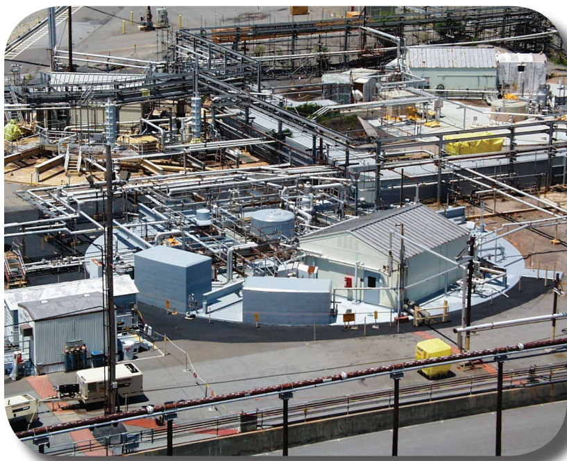
Looking down on the waste tank top of Tank 16
