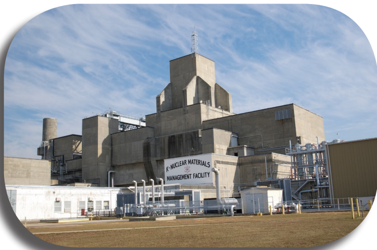
The K Area Materials Storage Facility (KAMS) is located in the building that housed K Reactor
