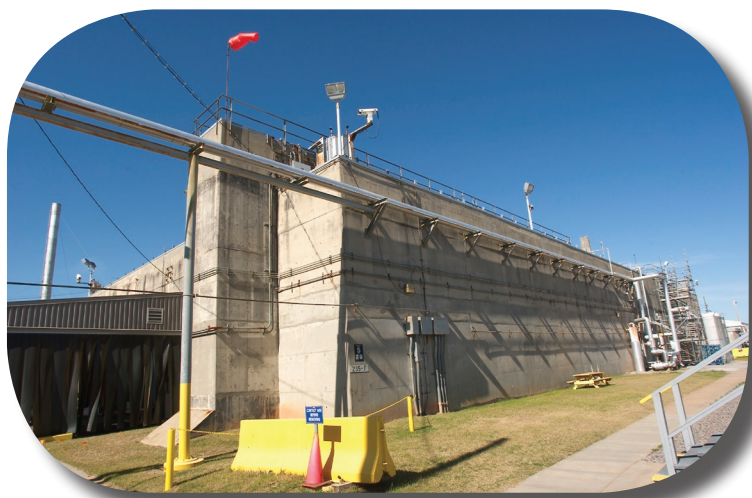
235-F Facility, future home of the 3013 Container Storage and Surveillance Capability Project
