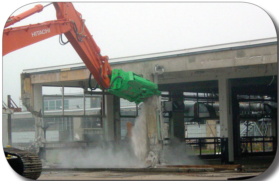
Building 313-M is one of more than 100 buildings demolished so far
