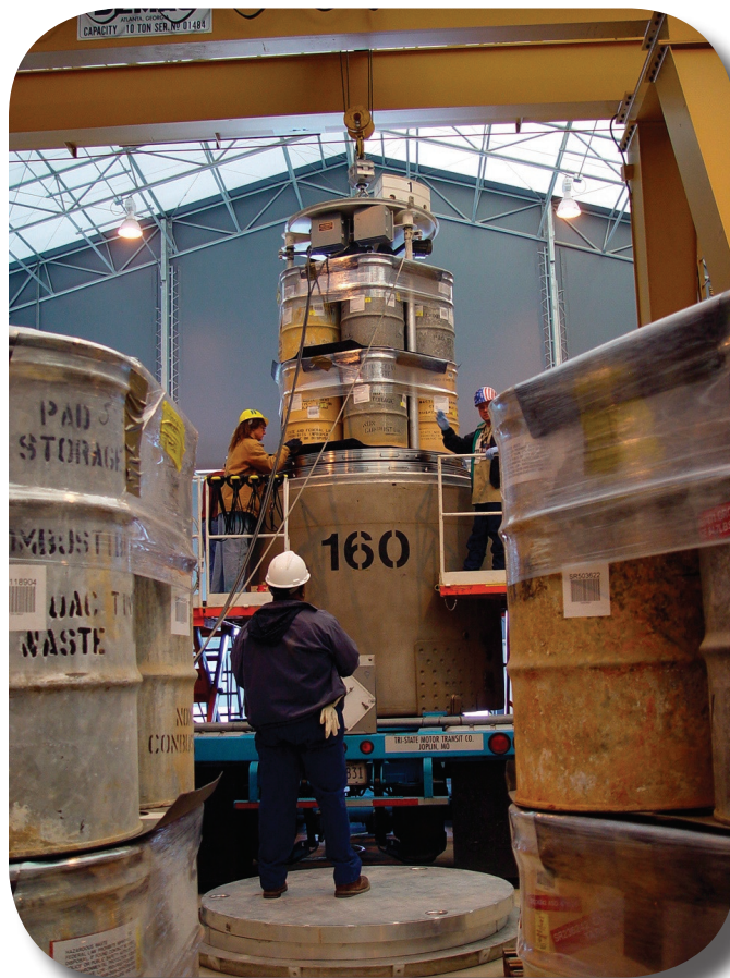
Loading TRUPACT II containers on TRU Pad 3 Burial Ground
