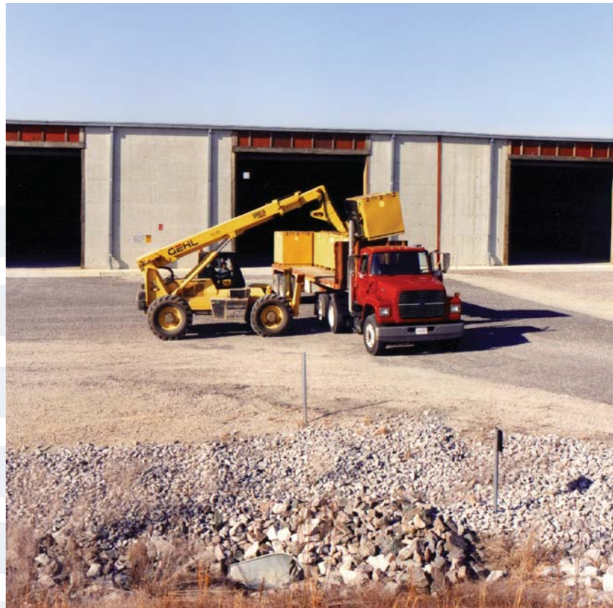
Low Activity Waste Vaults provide safe disposal for certain types of solid low-level waste.
