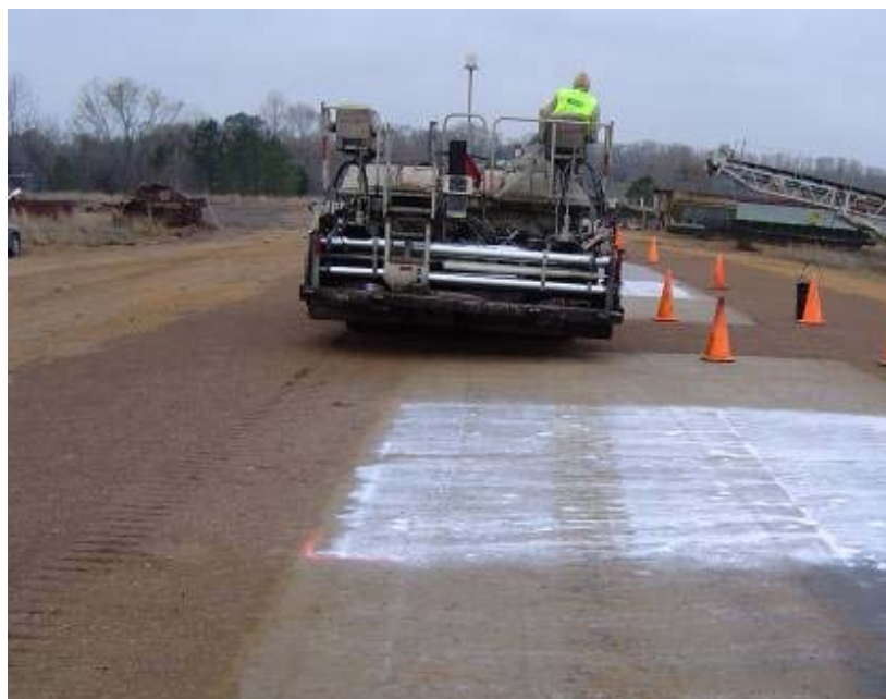
Figure 3-1. Application of construction traffic to a 2-day old CTB surface.
