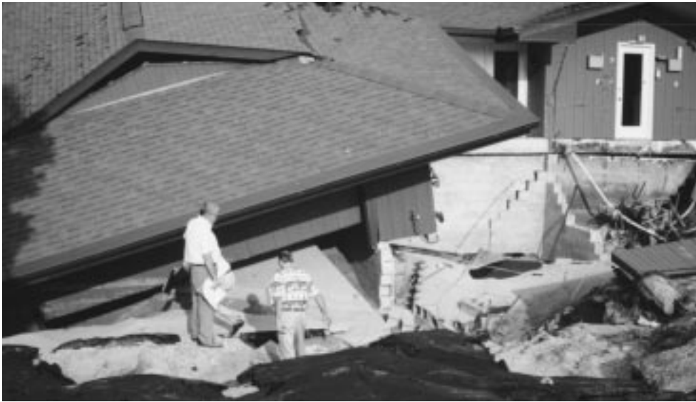
Flash flooding in Sheboygan County undermined the foundation of this house causing it to collapse.
