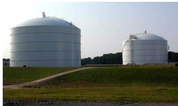
Cove Point Import Terminal, Maryland Photo courtesy of Dominion © 2003, http://www.dom.com
