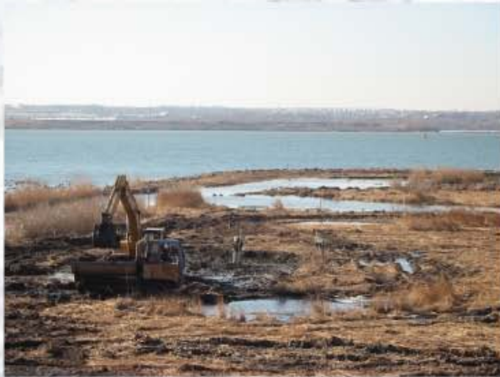
Construction of a new wetland.
