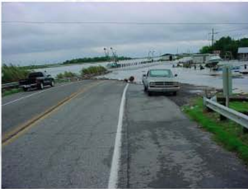
Evacuation route flooded from storm surge.
