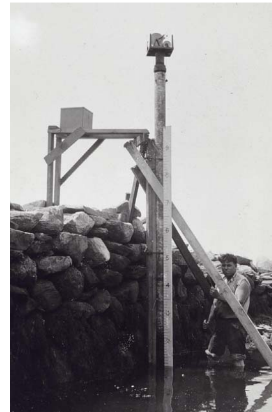
Portable tide gauge installation with tide staff
