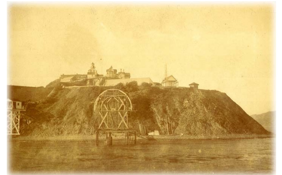
Construction of an early visual Tide Elevation Recorder at Alcatraz Island
