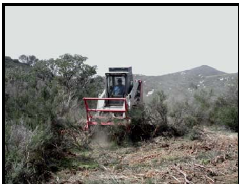
Figure 2 Mastication work at Poppet Flat
