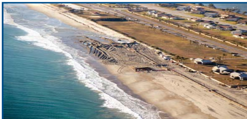
Aerial view of the Patrick Air Force Base, Florida beach nourishment project
