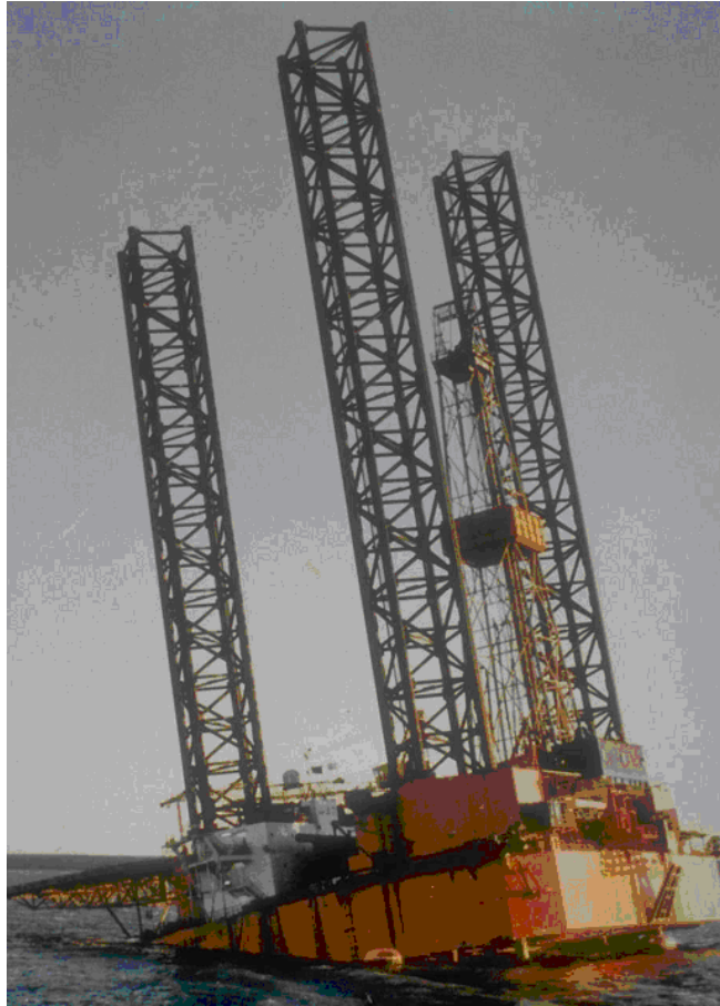
Figure 36: Rio Colorado rig photo to illustrate the robustness of the Levingston III design to leg settlement.
