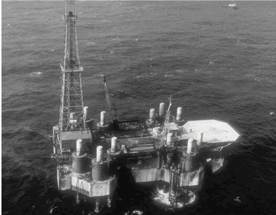
Figure 40: Mr Louie First Jackup built to Class Rules.
