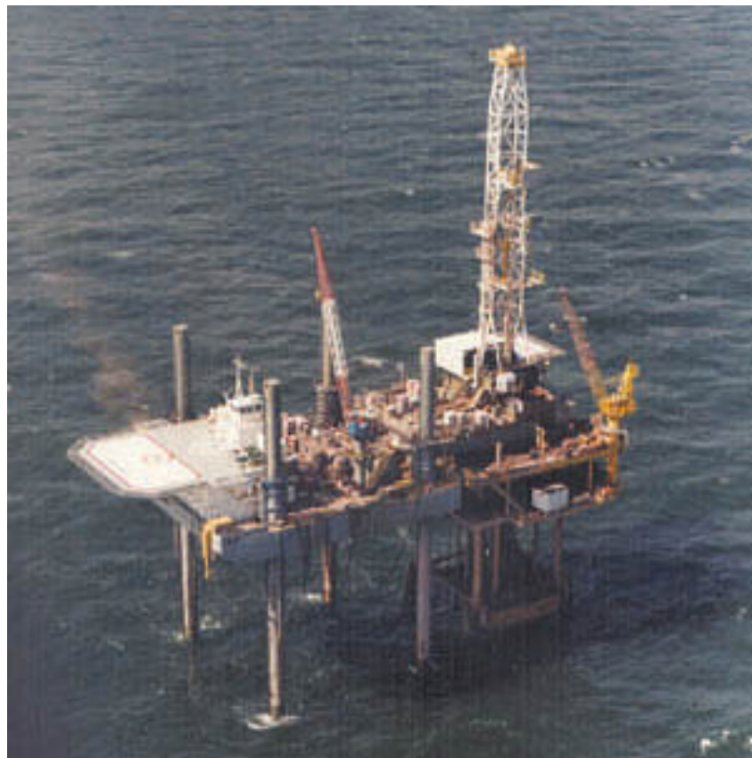
Figure 17: Nabors Dolphin 105 on location working at a fixed platform.
