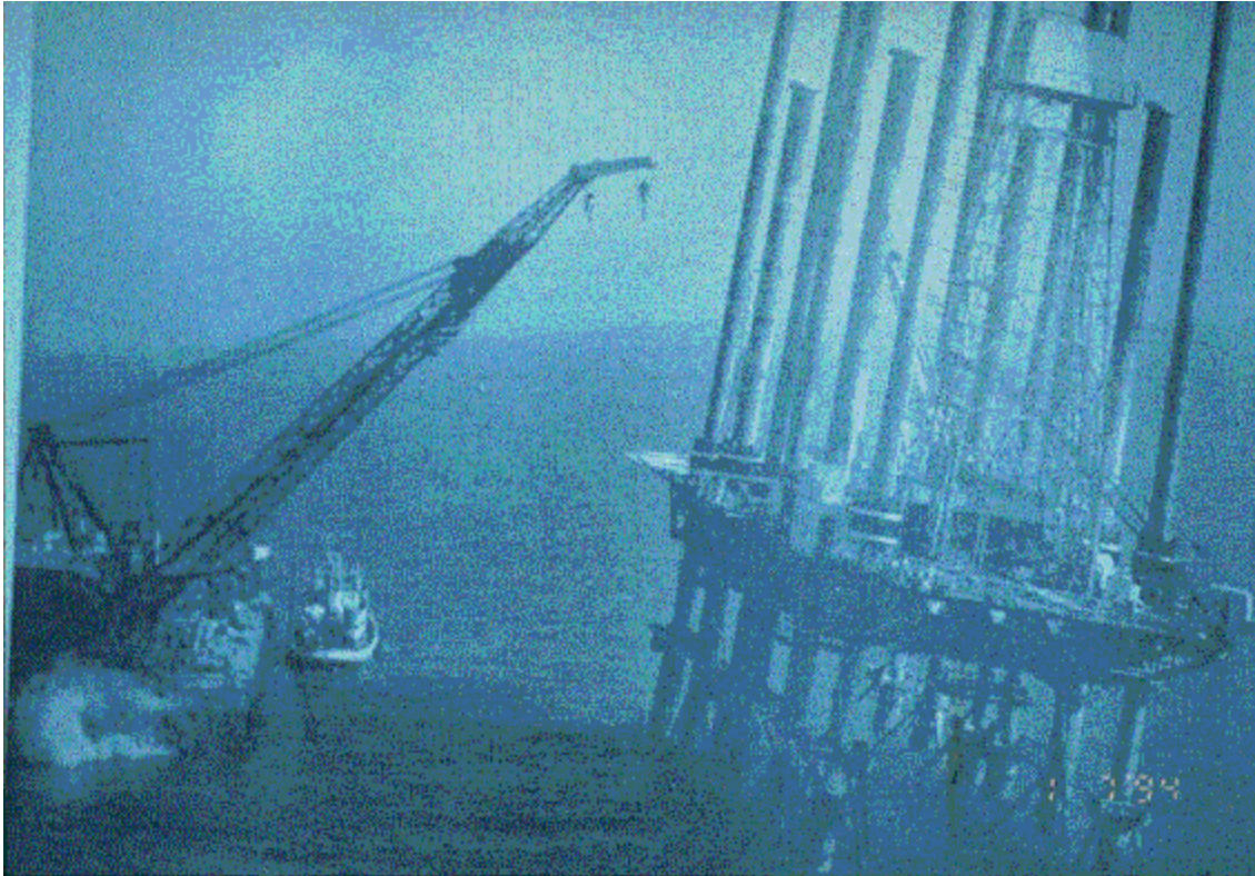
Figure 41: Mr Gus settled on location – prior to preload requirement
