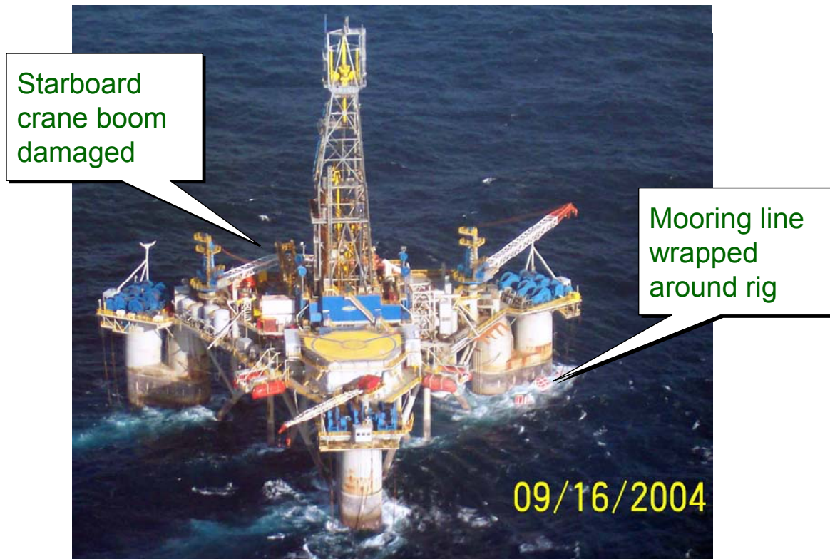
Figure 14: Noble Jim Thompson with damages noted.
