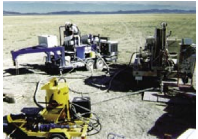
The microhole drilling system is shown here in central Nevada drilling cased 1.25-inch diameter microholes for emplacement of seismic instrumentation. The tan equipment (right) is the coiled tube drilling rig, the blue is a mud conditioning system, and the yellow is a PVC casing grouting system.
