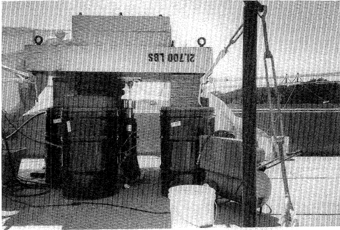
Fig. 17. The Sandia shaker in place on the I-40 Bridge.
