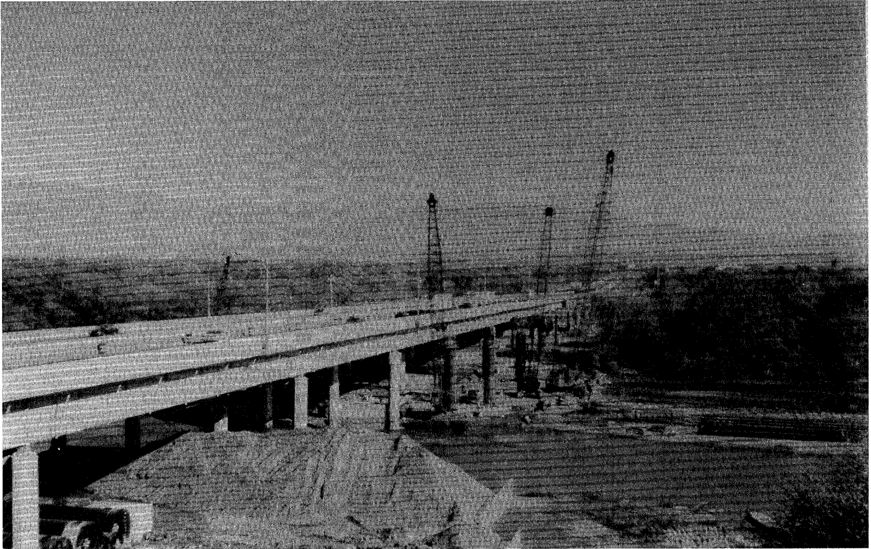
1. I-40 Bridges over the Rio Grande in Albuquerque, New Mexico.
