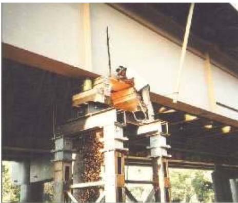
(a) Introduction of damage in one of the bridge girders by electric saw cutting
