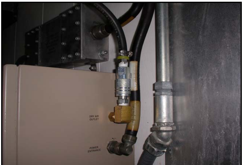
Photo 3: Quick disconnect replacement
