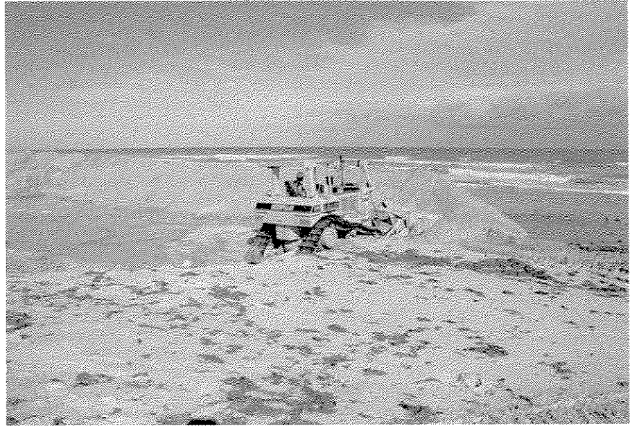
A bulldozer moves sand in a beach restoration project in Florida
