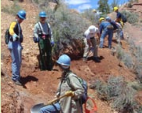
Trails Unlimited providing on-the-job trail construction training on Utah's Dixie NF.
