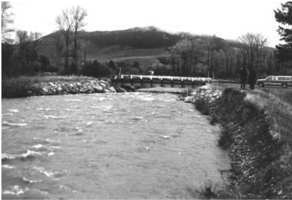
Figure 13—Vigilante Bridge, Beaverhead-Deerlodge National Forest. This 40 foot bridge constricts the channel and has caused upstream aggradation and contraction scour through and below the bridge.
