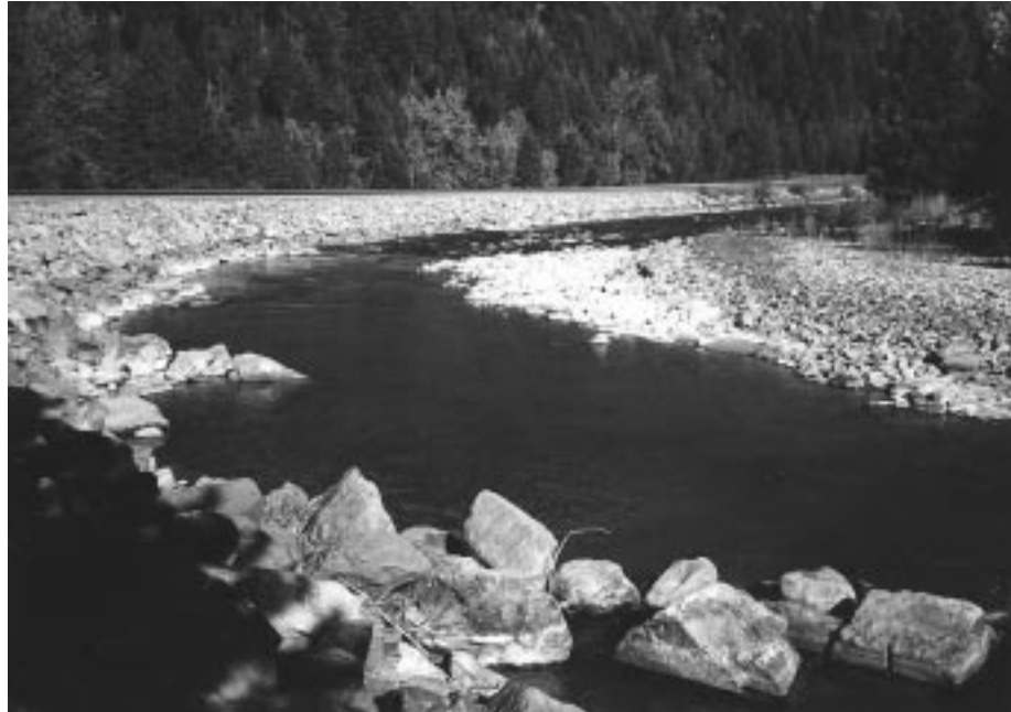
Figure 17—Fisher River Bank Stabilization, Kootenai National Forest. Use of rock vanes to protect the stream bank from scour.
