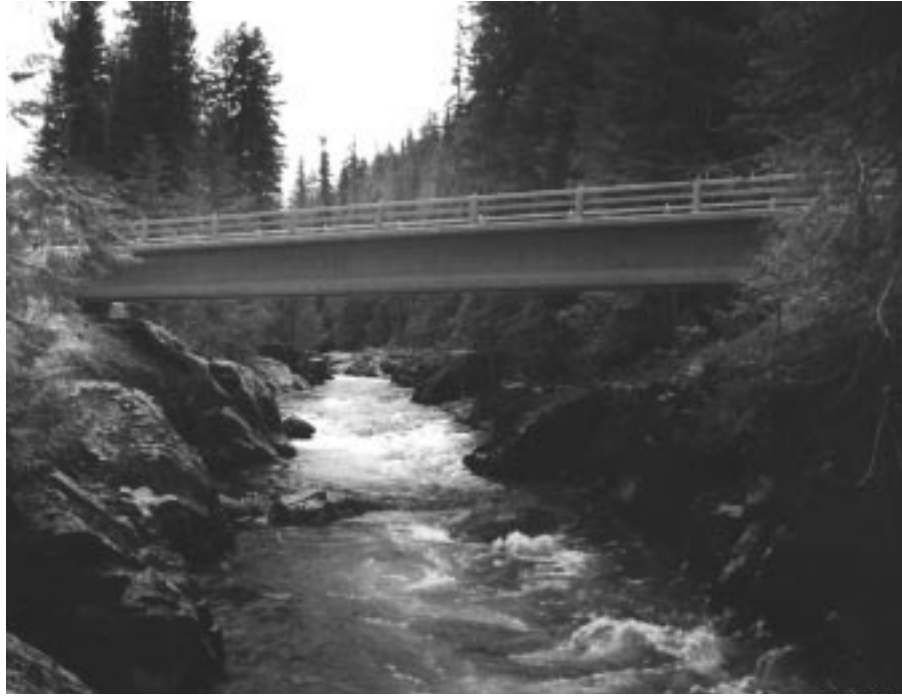
Figure 5—Libby Creek Bridge, Kootenai National Forest. Bridge footings are set into non-erodible bedrock as well as being outside the channel and well above flood waters. Bridge is categorized as Low Scour Risk.
