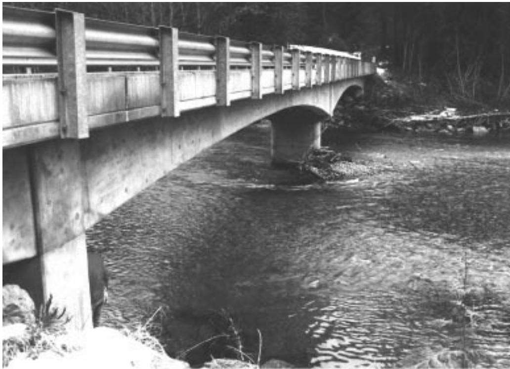
Figure 14—Irene Bridge over Cascade River, Mt. Baker - Snoqualmie National Forest, Region 6. Drift build-up on upper side of pier.
