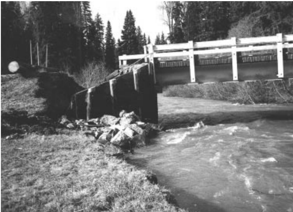
Figure 15—Monture Bridge, Lolo National Forest. An example of abutment fill failure with little damage to the bridge.
