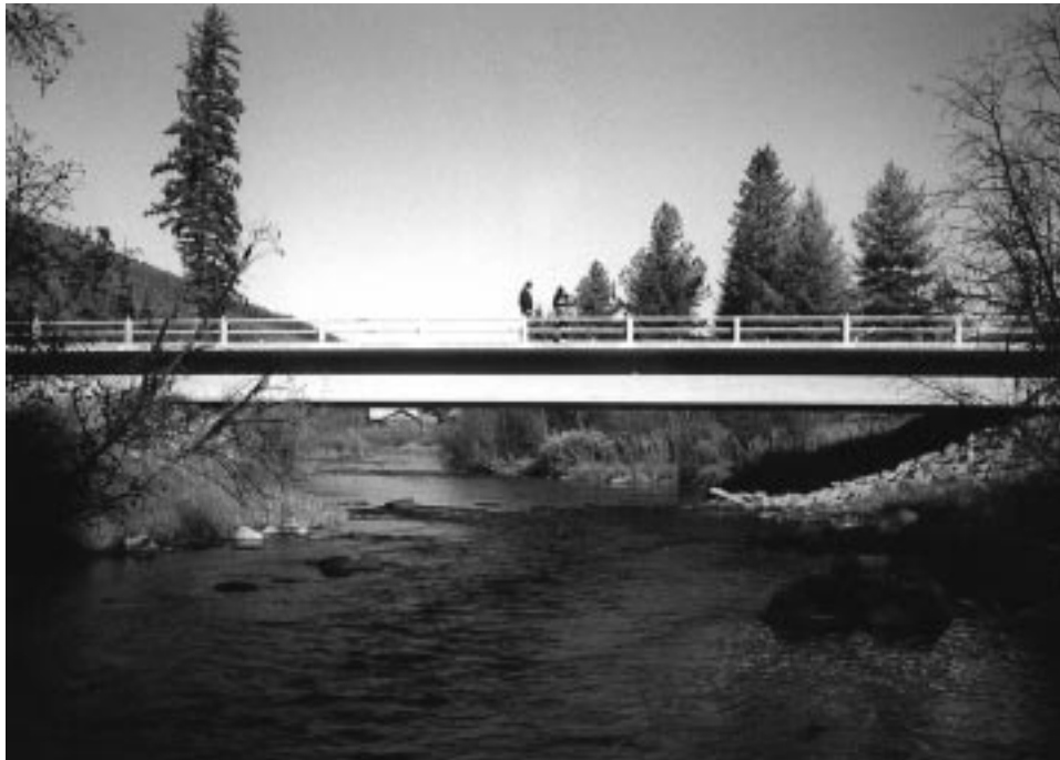
Figure 10—Independence Creek Bridge, Idaho Panhandle National Forest. Example of a spill through (trapezoidal) abutment configuration. See Figure 9 for an example of a vertical wall abutment with wingwalls.
