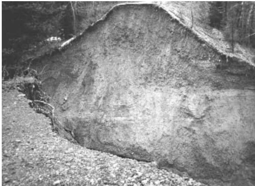
Figure 8—Moss Creek, Idaho Panhandle National Forest. Piping and subsequent scour of this culvert resulted in failure of the entire fill introducing a large amount of sediment into the stream. With Step 1b, Management Priority Analysis, the potential for resource damage at similar sites could be considered as unacceptable.
