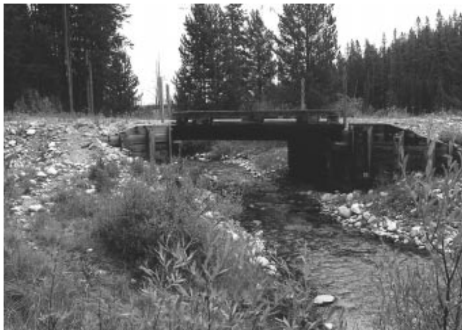
Figure 9—LaMarche Creek Bridge, Beaverhead National Forest. Typical single-span, treated timber bridge supported on vertical wall abutments, with wingwalls, on mudsills crossing a mountainous stream.
