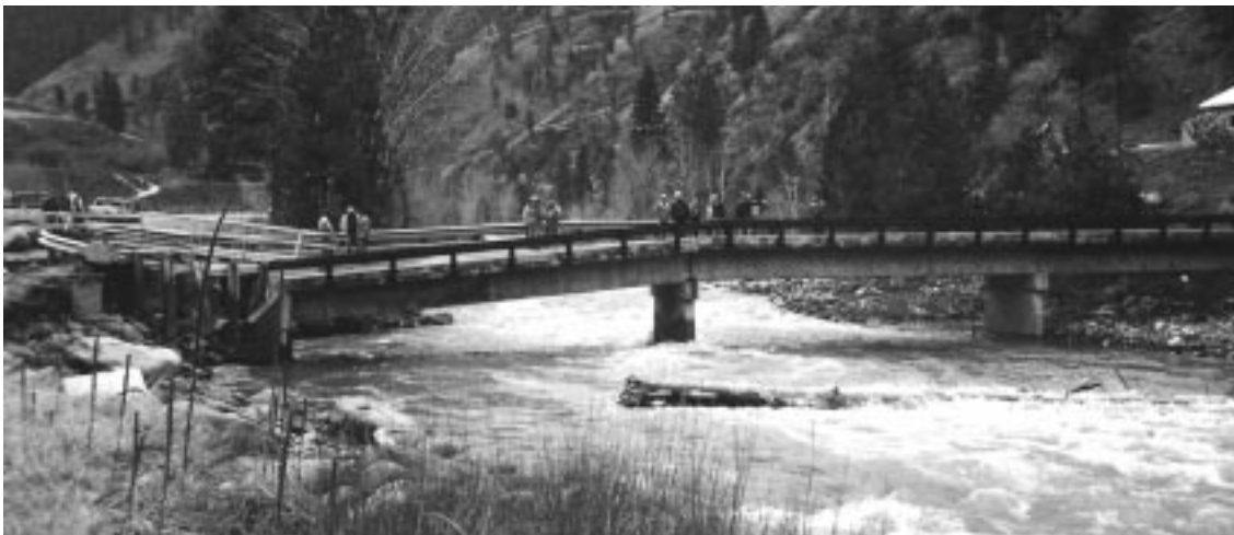
Figure 1—Little Salmon River Bridge, Nez Perce National Forest. A January 1997 flood event scoured the abutment and one of the intermediate piers causing failure.
