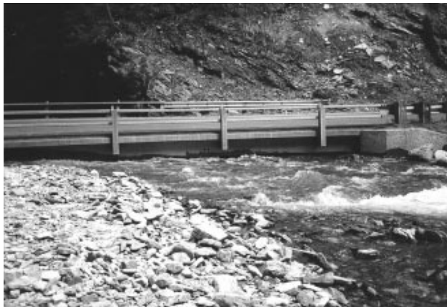
Figure 11—Eagle Creek Bridge, Idaho Panhandle National Forest. Backwater effects from the main river caused aggradation at the mouth of this tributary and inadequate clearance for the bridge. Note, the following year the tributary flushed and the stream re-established the normal channel depth.
