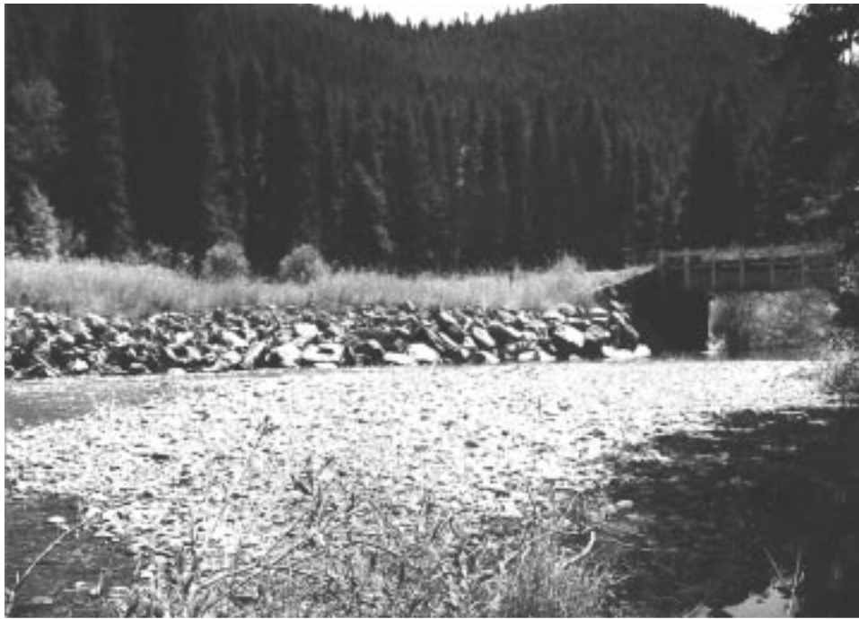
Figure 16—Monture Bridge, Lolo National Forest. Repair of abutment fill failure and use of riprap as a scour countermeasure.
