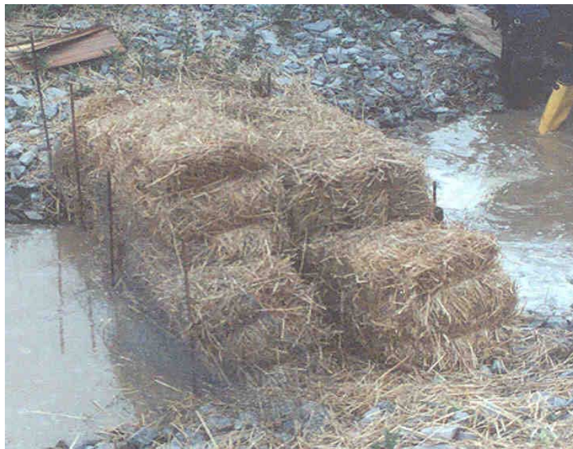
Figure 4-29. Hay filter barrier.
