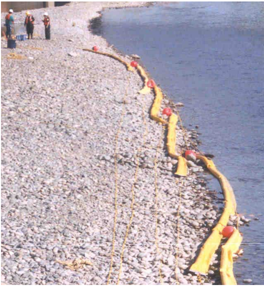
Equipment is deployed along shore.
