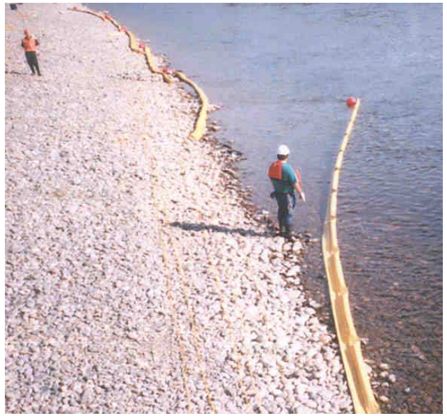
First boom is deployed.
