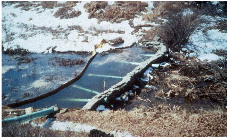
Figure 4-23. Underflow dam with debris boom.
