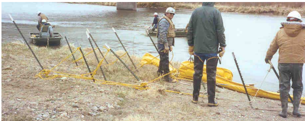
Figure 8-9. Multiple booms being anchored (DOWCAR, 1997).
