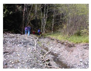
Looking upstream at newly constructed diagonal ditch. This is a small portion of the ditch that is proposed to be filled in. Person on right is at the approximate elevation of the existing floodplain. Newly graded area is on the left.
