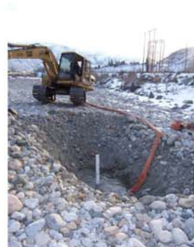
Typical test hole showing excavator, staff gage and suction hose.
