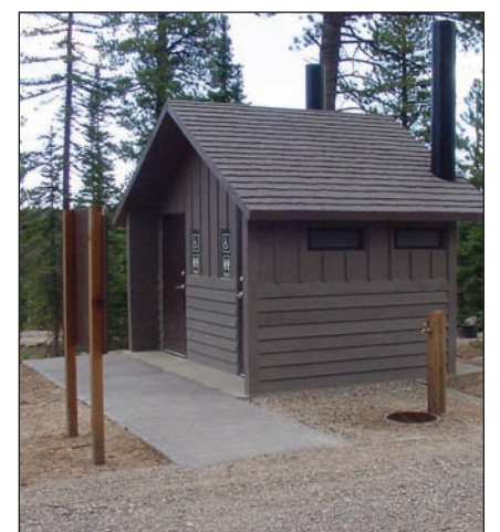
This toilet is typical of those installed during the rehabilitation of DeMotte Campground on the North Kaibab Ranger District. The rehabilitation was completed in 2006.
