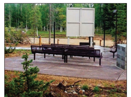
A new barrier-free amphitheater was constructed at Demotte Campground; part of the renovation project completed in 2006.
