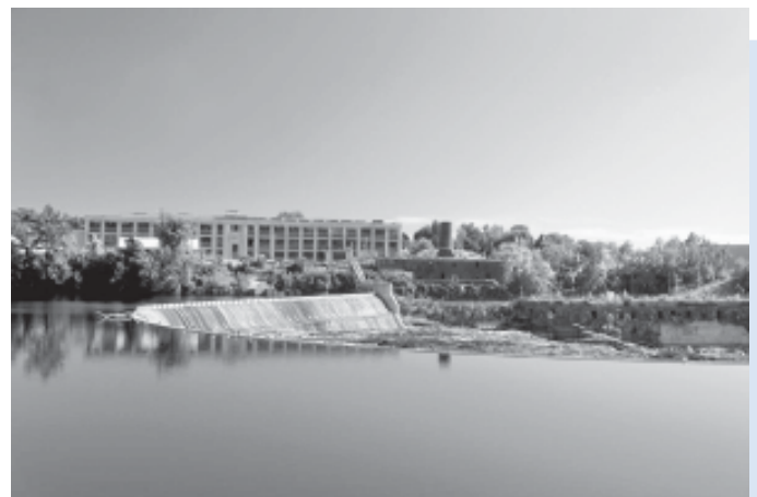
GE Hudson Falls Plant Site and Allen Mills
