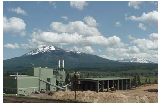
Figure 21. Burney Forest Power stand-alone powerplant.
