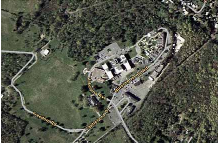
Figure 6: A diagram of the aerial photograph of the primary building cluster on the Castle Point campus
