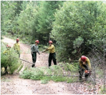
A crew clears vegetation from the roadway as part of on-going road maintenance activities.
