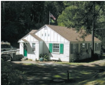
The Forest has a number of 1930s era CCC historic buildings such as this former ranger residence.
